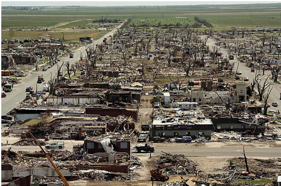
FIGURE 1-4 Greensburg, KS, May 16, 2007 — The center of town 12 days after it was hit by an F5 tornado with 200mph winds. Debris removal is moving at a record pace, but reconstruction will likely take years. (Photo by Greg Henshall/FEMA News Photo)
