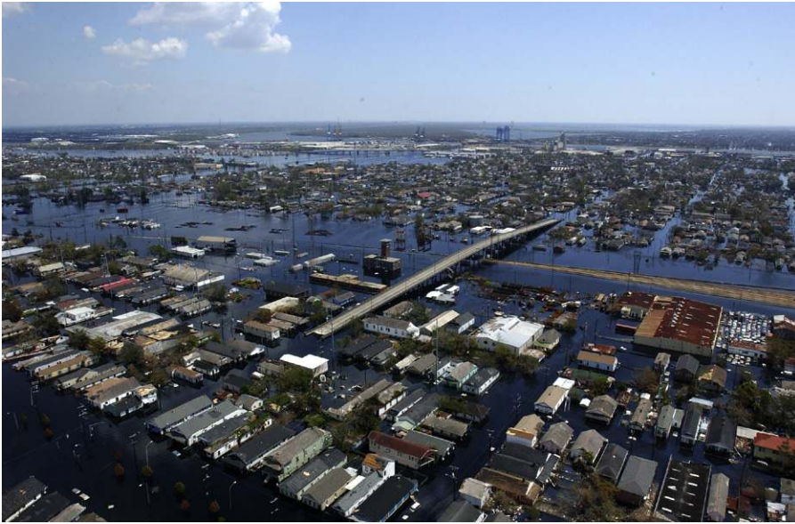
FIGURE 1-2 New Orleans, LA, September 8, 2005 — Neighborhoods and roadways throughout the area remain flooded as a result of Hurricane Katrina. (Photo by Jocelyn Augustino/FEMA News Photo)
