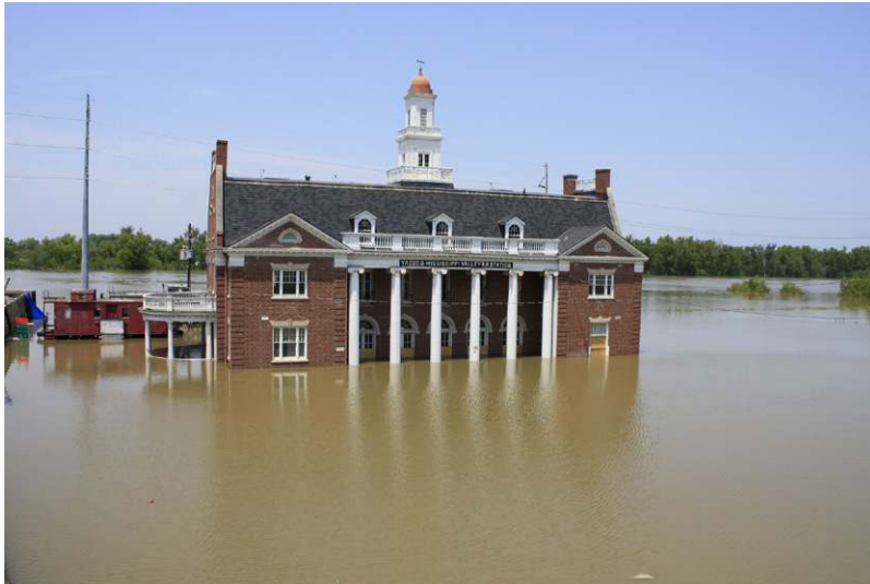
Vicksburg, MS, May 12, 2001 – The lower floor of the historic Yazoo Mississippi Valley Railroad Station, which is located in Vicksburg, Mississippi, is submerged by the rising Mississippi River. FEMA is working with local, state, and other federal agencies to assist residents affected by the floods. (Photo by Howard Greenblatt/FEMA)
