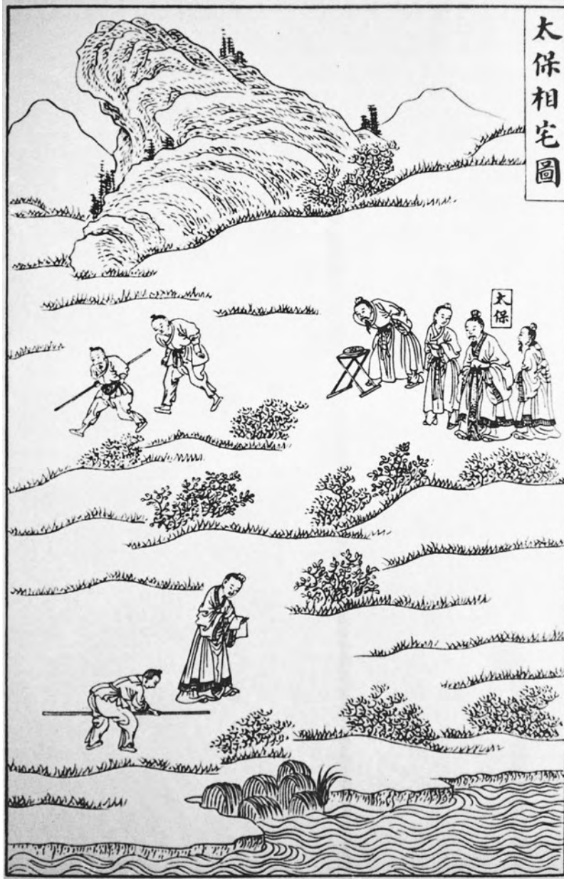
Fig. 7.2. Chinese geomancer. Prior to laying out a new city, an expert geomancer or fēng-shui master consults a compass-like device to ascertain the flow of energy ( chi ) in the locale. He will then use his readings to situate artificial structures in harmony with their natural surroundings.
