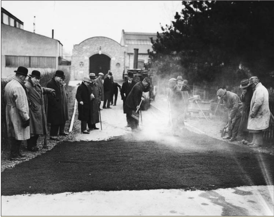
This section of road was improved by building a tarmac surface early in the twentieth century.
