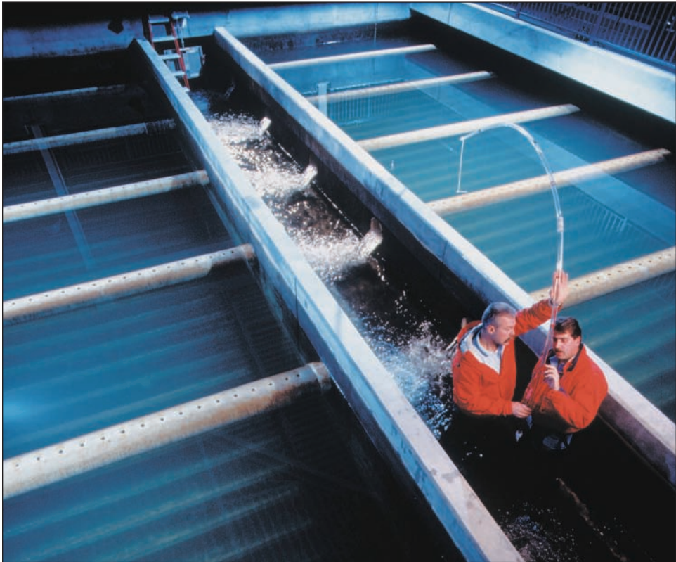
At a water-treatment plant, two sanitation technicians take a sample of the water so it can be tested.
