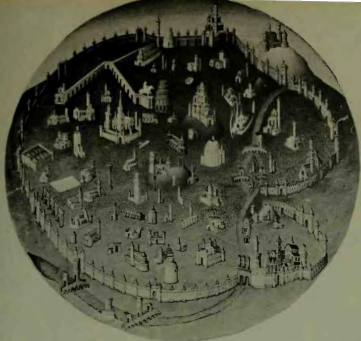
Plan of Rome. Fifteenth-century miniature, from the "Très riches heures du duc de Berry," by Pol Limbourg. Chantilly Museum
