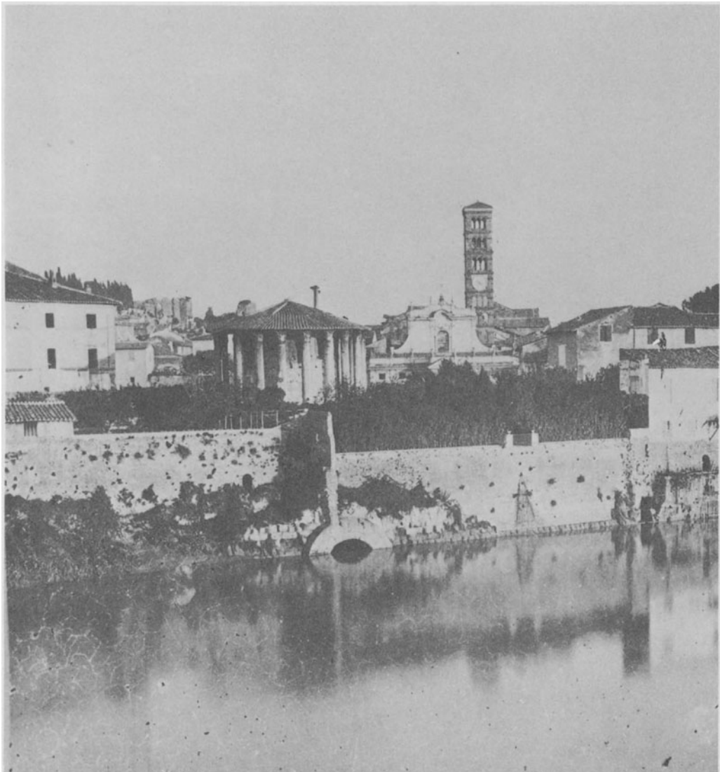
30.4 The arched Cloaca Maxima, discharging into the Tiber.
