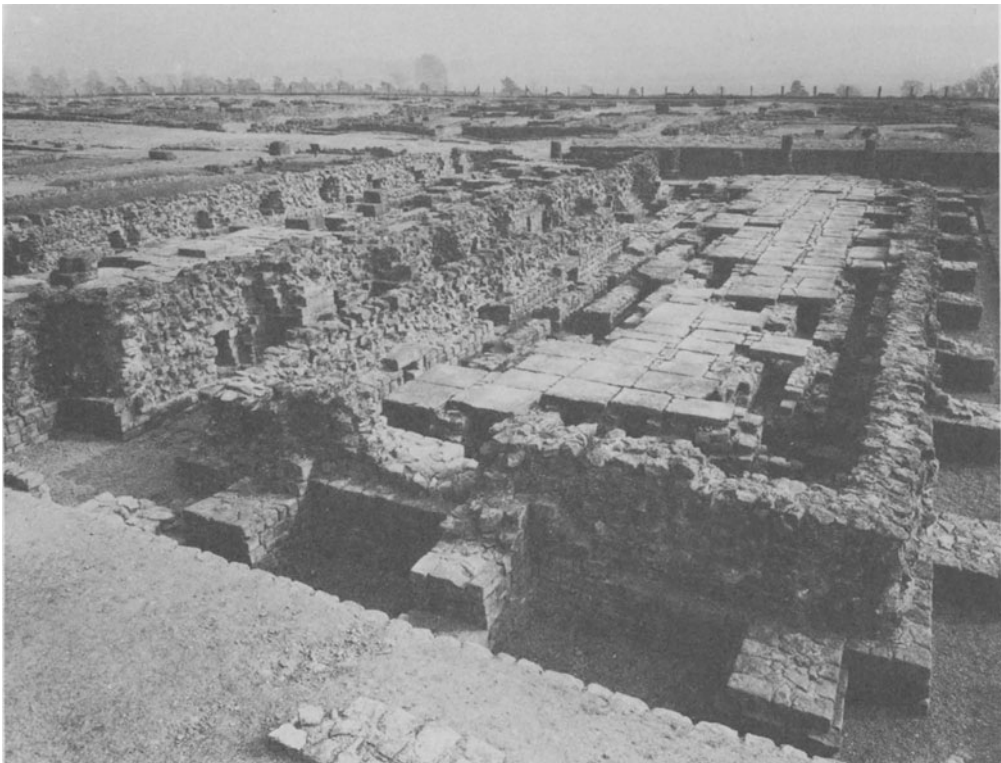
38.9 The granaries at the Roman military post at Corstopitum (near Corbridge, Northumberland), which were built by Severus and his sons, c. A.D. 205.
