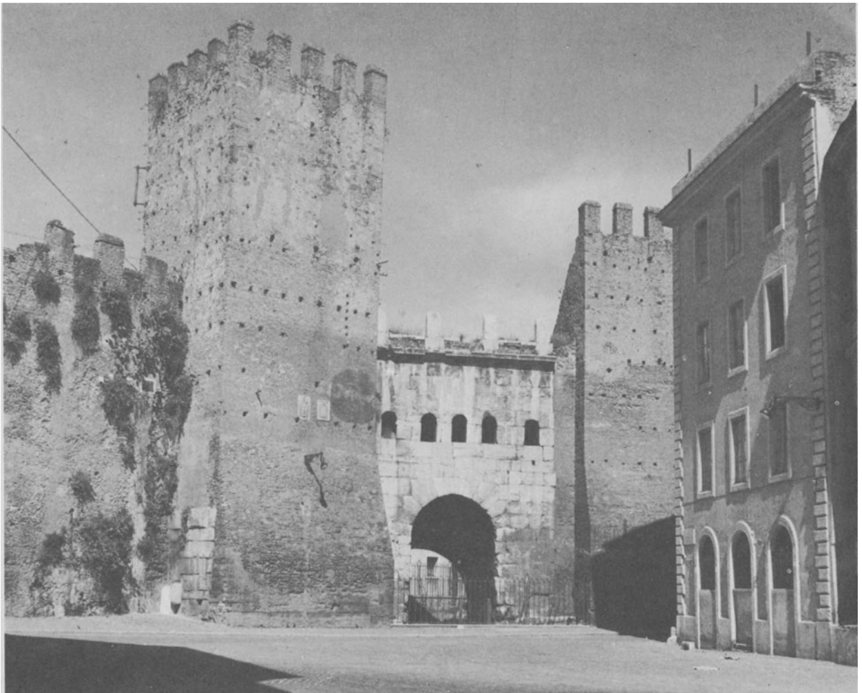
32.8 Porta Tiburtina. The outer side. The earlier Augustan arch was incorporated in the Aurelian Wall as a gateway. Honorius added a second outer arch and rectangular towers.
