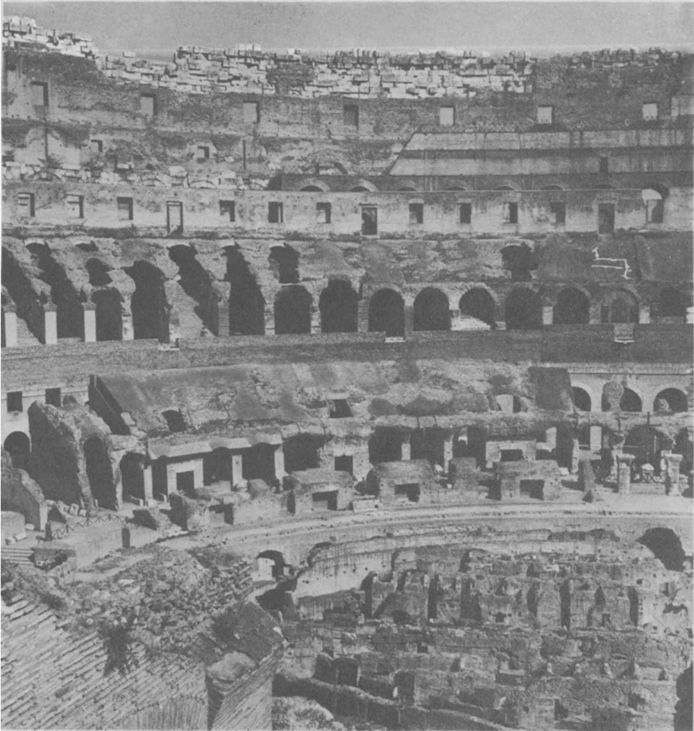
36.5 The Colosseum. Internal view. The masonry in the bottom right-hand side of the picture was below the wooden floor of the arena.
