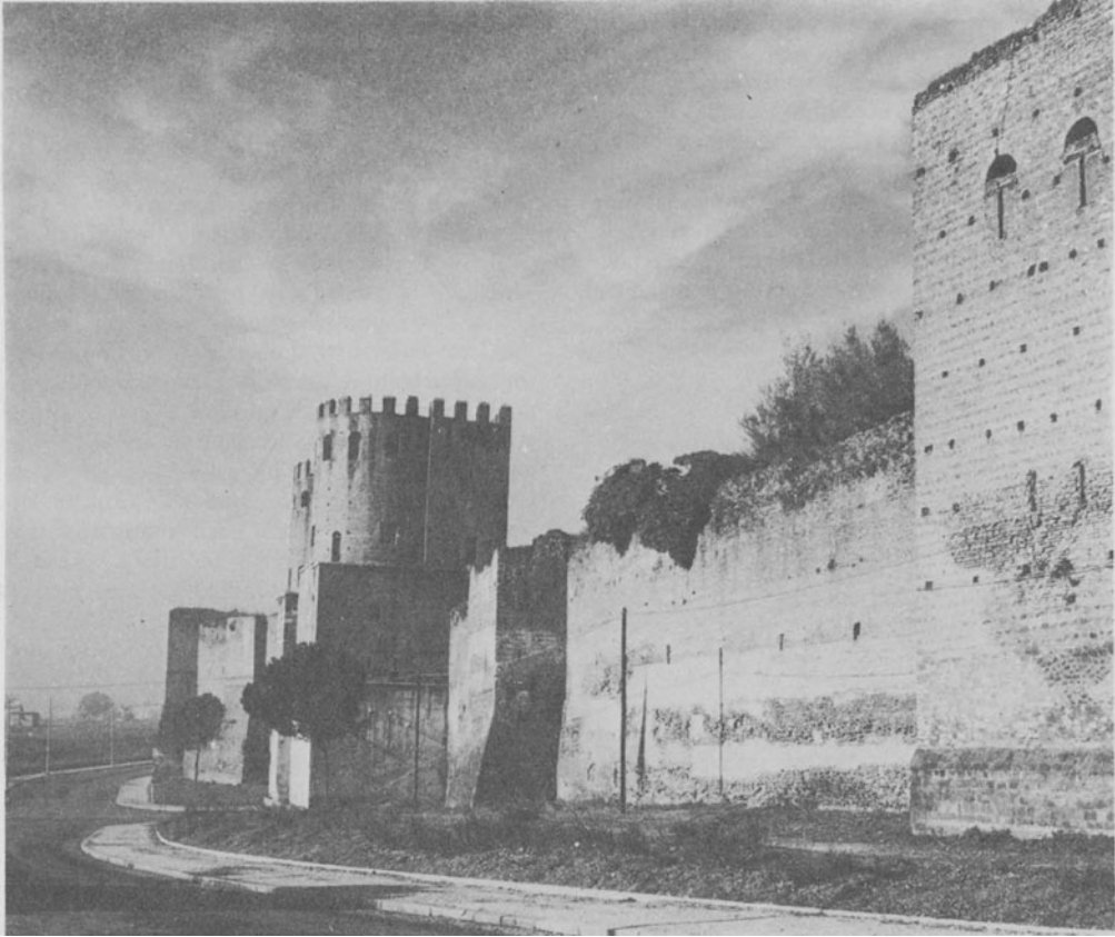
41.11 Aurelian's Wall at Rome, near the Porta Appia. Built of concrete, and faced with brick, the Wall is some 12 miles long and has 381 towers.
