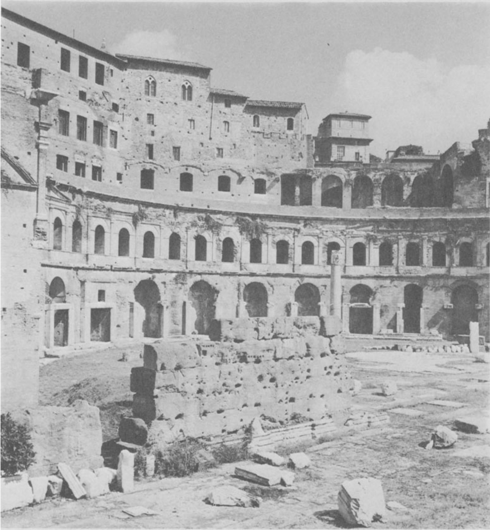
39.13 Trajan's Market (Mercatus). This market complex contained 150 shops ( tabernae ) and a two-storeyed hall. Streets at the back provided access to the building at three different levels.
