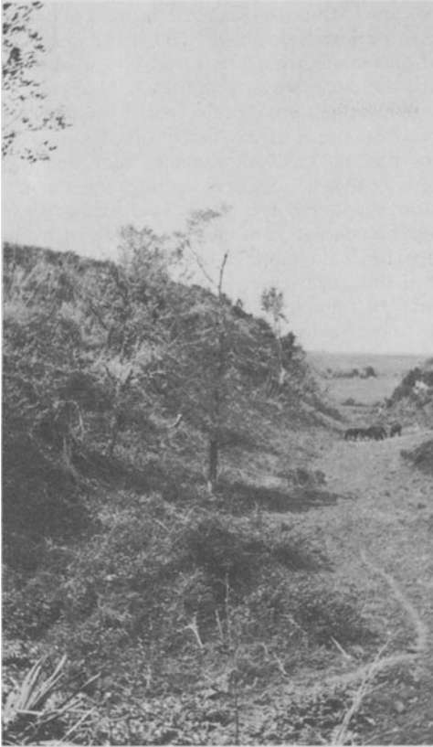
5.10 Early earthworks at the Latin town of Ardea. They show the kind of agger that protected the exposed parts of Rome in the Regal period.
