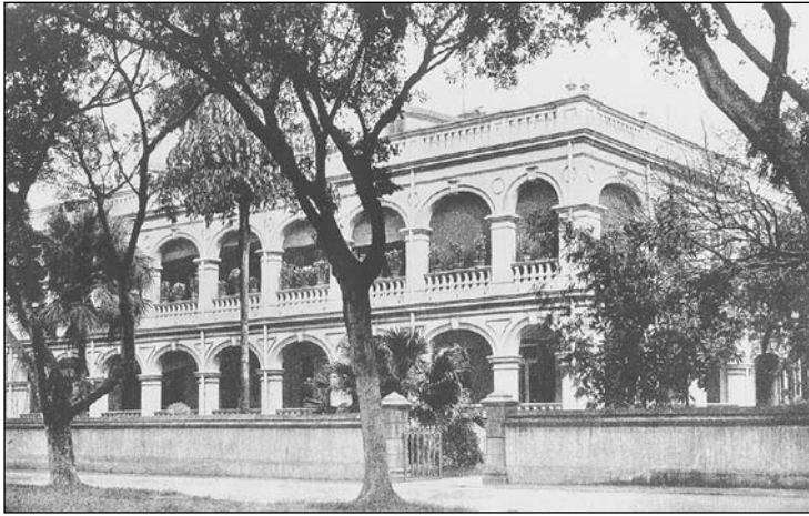
The treaty-port style. Its Anglo-Indian origins are apparent: thick walls, deep verandas on all sides, and vaguely Corinthian style, but open to whatever breezes can help to ease the hot climate. This is the office of an American firm in Guangzhou. (From Arnold Wright, Twentieth Century Impressions , London, 1908, p. 792)
