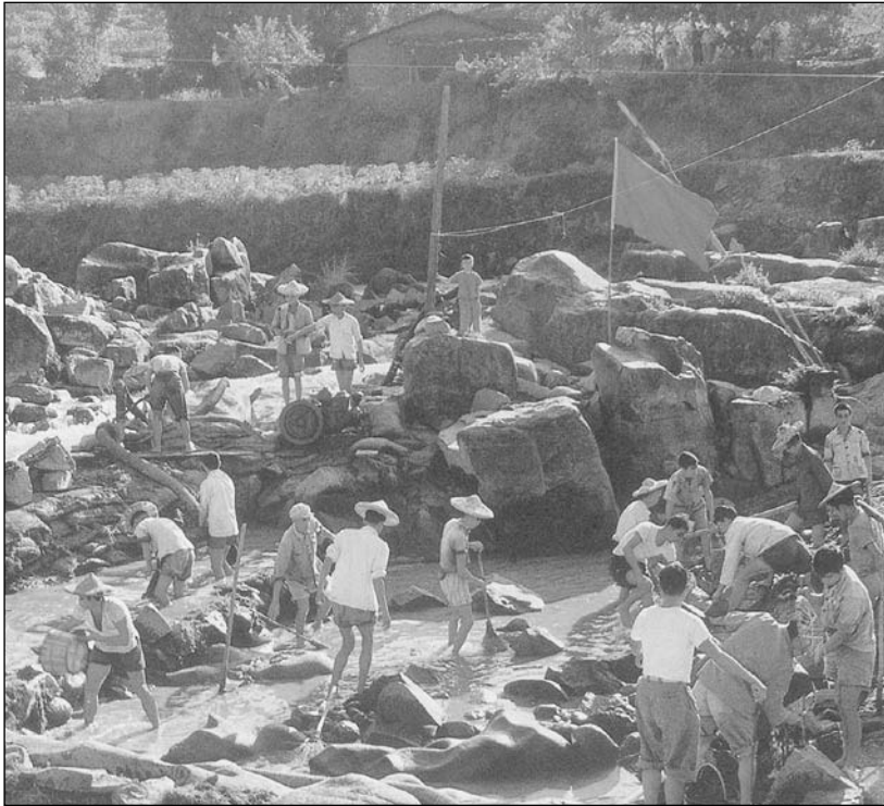
The mass line in action: some of the 100,000 people involved in building, largely by hand, a new irrigation dam outside Beijing. This is in fact an ancient system; similar armies of mass labor built the Great Wall, the Grand Canal, and other monumental public works in the long past. (R. Murphey)
