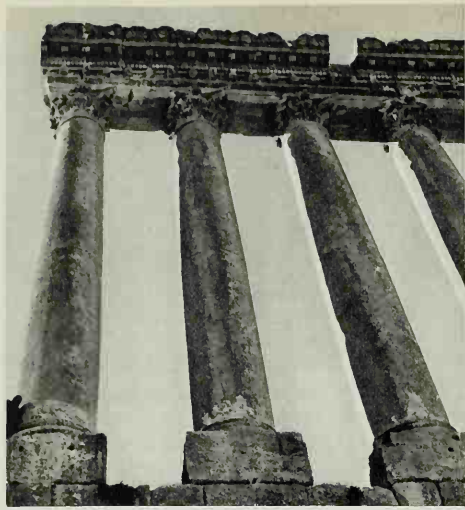
644. ROMAN ART IN ASIA. Column of the temple of Jupiter Heliopolitanus at Baalbek (Lebanon). Originally there were fifty-four columns, which at 65 feet high are among the tallest in the world. 1st-2nd centuries A.D.
