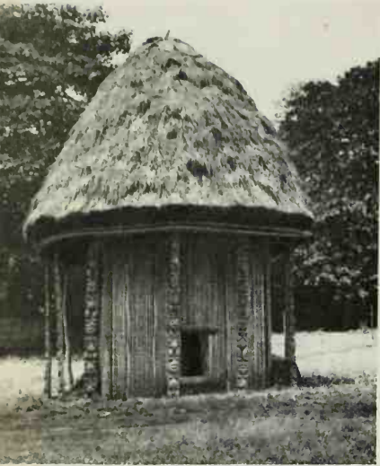
117. BAMILEKE. CAMEROONS. Hut with carved columns.
