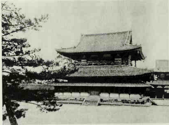
724. JAPANESE. ASUKA. The Kondo (Golden Hall) of the Horyuji, near Nara. End of the 6th century—beginning of the 7th century A. D.
