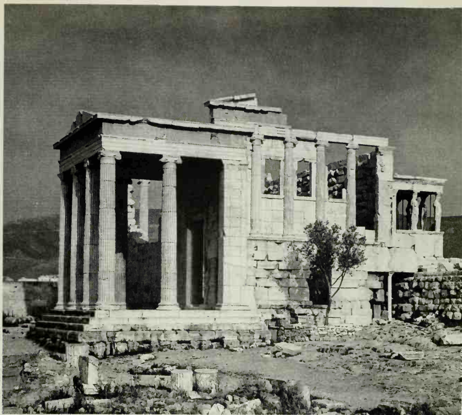
428. GREEK. IONIC. The Erechtheum on the Acropolis, Athens. Beginning of the 5th century B.C.
