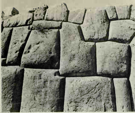
142. CENTRAL ANDES. PERU. Detail of the walls of Sacsayhuaman.
