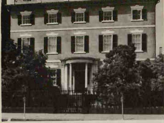
197. U.S.A. FEDERAL. SAMUEL McINTIRE (1757-1811). Gardner-White-Pingree house, Salem, Massachusetts. 1804-1805.
