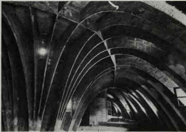
682. SPAIN. ANTONI GAUDÍ (1852–1926). Loft of The Casa Milá, Barcelona. 1905–1910.
