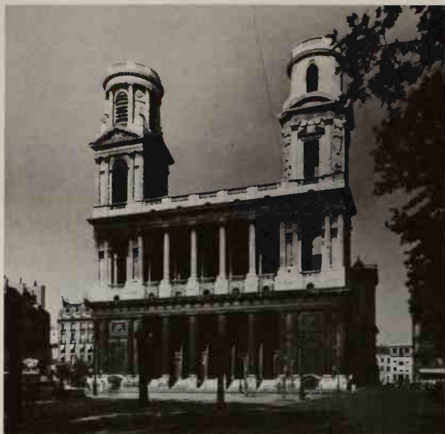
42. FRANCE. J. N. SERVANDONI (1695–1766). Façade of St Sulpice, Paris. 1733–1749. Church begun in 1646; north tower rebuilt by Chalgrin, 1777.
