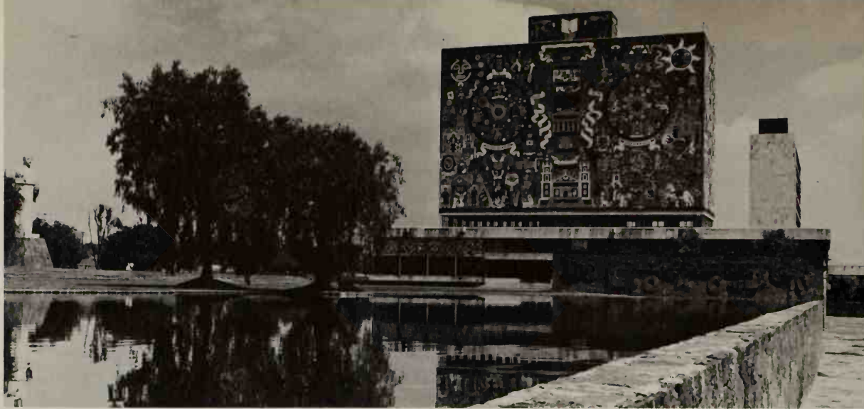
1154. MEXICO. O'GORMAN, SAAVEDRA and MARTINEZ DE VELASCO. Central library, University City, Mexico City. 1951-1953.
