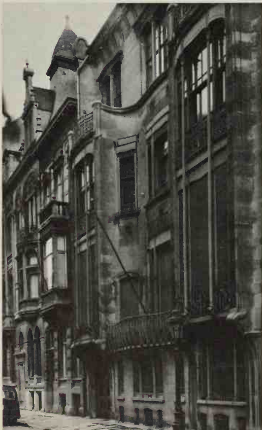
957. BELGIUM. VICTOR HORTA. Solvay house, Brussels . 1895–1900.
