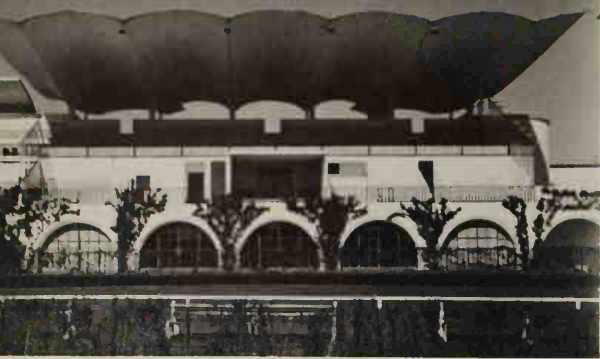
949. SPAIN. EDUARDO TORROJA (1899–1961). Grandstand at the Zarzuela racecourse, near Madrid. 1935.
