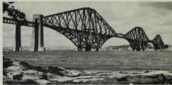
573. BRITAIN. The Firth of Forth railway bridge. 1882–1889. Constructed by Sir John Fowler and Sir Benjamin Baker.
