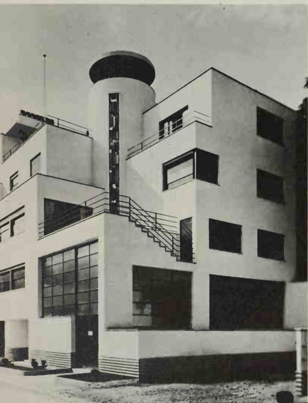
677. FRANCE. ROBERT MALLET-STEVENS (1886–1945). House in the rue Mallet-Stevens, Paris. 1927.
