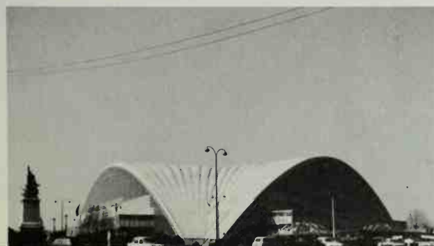
684. FRANCE. BERNARD ZEHRFUSS (b. 1911). Centre National des Industries et Techniques, Paris. Built in collaboration with R. Camelot and J. De Mailly. 1958.
