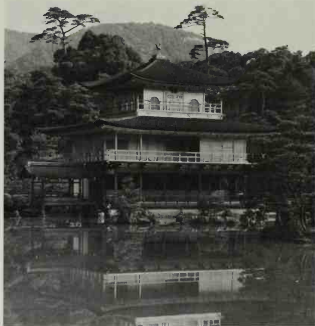
282. JAPAN. Kinkakuji ('golden pavilion') at Kyoto. Built 1397 for Ashikaga Yoshimitsu. Muromachi period.
