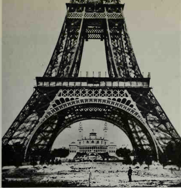
680. FRANCE. GUSTAVE EIFFEL (1832–1923). The Eiffel Tower in Paris in the course of construction in 1888. Completed 1889.
