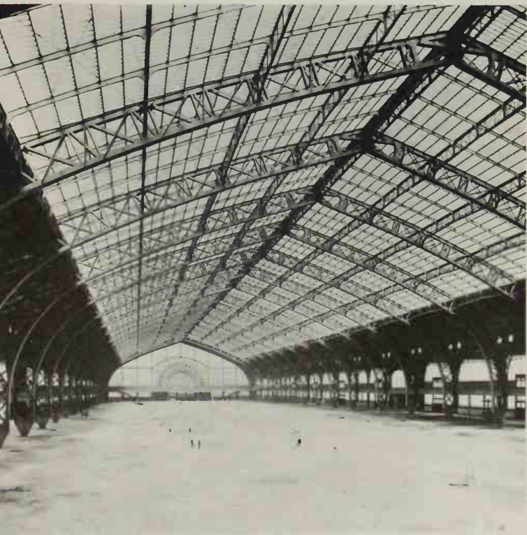
413. FRENCH. The Machinery Hall constructed in Paris for the International Exhibition of 1889 by the architect F. Dutert (1845–1906) in collaboration with the engineer Victor Contamin (1840–1893). Height 150 feet, length 1400 feet, span 370 feet.
