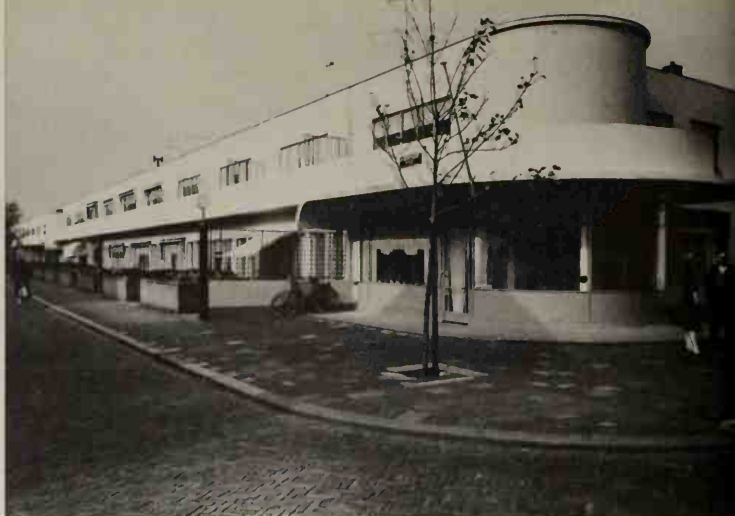
968. HOLLAND. J. J. P. OUD. Workers' housing estate, Hook of Holland. 1924–1927.
