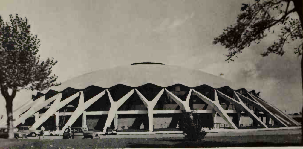
934. ITALY. PIER LUIGI NERVI (b. 1891). Palazzetto dello Sport, Rome (with A. Vitellozzi). 1959.
