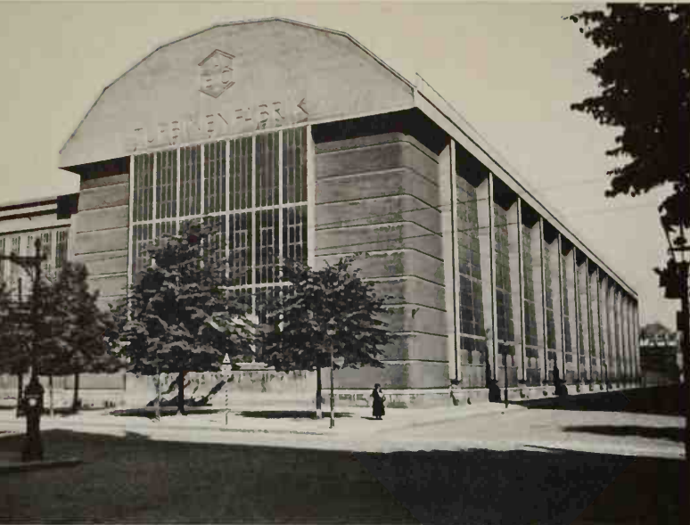
736. GERMANY. PETER BEHRENS (1868–1940). AEG turbine factory, Berlin. 1909.
