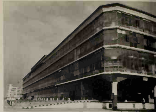
978. BRITAIN. E. OWEN WILLIAMS (b. 1890). Boots' factory, Beeston, near Nottingham. Completed 1932.
