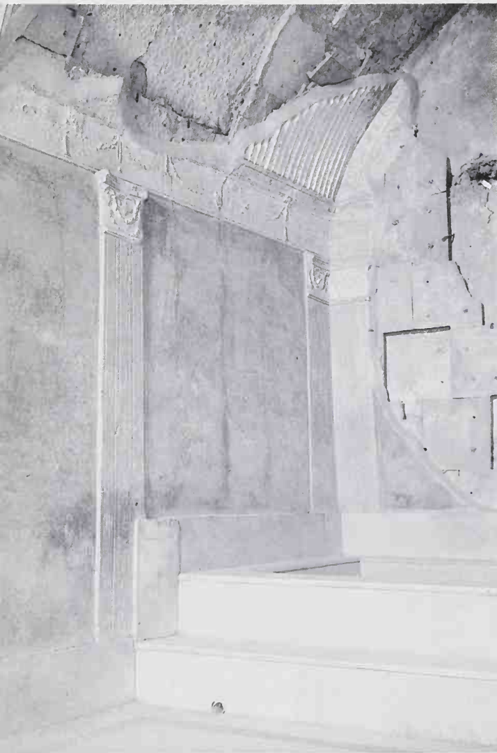
17 Interior view of the Stabian Baths, Pompeii This is a particularly interesting example of how marble sheeting and stucco decoration were applied over the brick understructure of most Roman buildings, achieving great delicacy in the slim pilasters, flower garlands and fluted decoration of the barrel-vault
