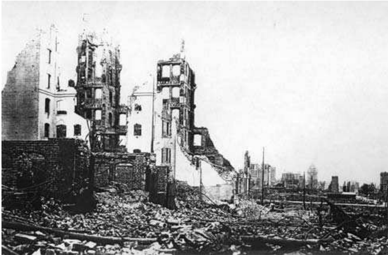
Earthquake damage in San Francisco, 1906. The quake, which killed 700, was the deadliest in U.S. history. Quakes of similar magnitude (8.3 on the Richter Scale) killed 25,000 in Mexico City in 1985 and 100,000 in Tokyo in 1923. Courtesy of the Library of Congress.
