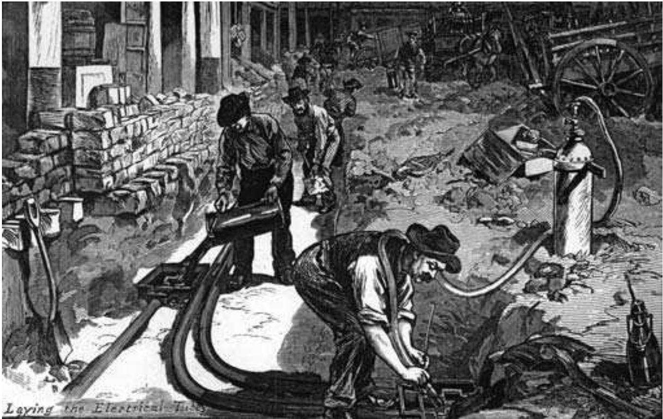
Laying the Electrical Tubs Laying electrical cables in New York, drawn by W.P. Snyder for the 28 June 1882 edition of Harper's Weekly . The enormous costs involved in "wiring" an area meant that customer-rich cities enjoyed electrical service long before isolated rural areas did. Courtesy of the Library of Congress.
