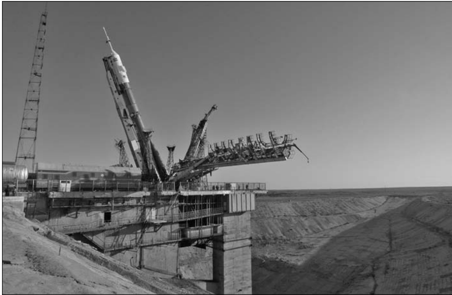
Figure 7-2: A Soyuz spacecraft and its launch vehicle being erected at the launchpad.
