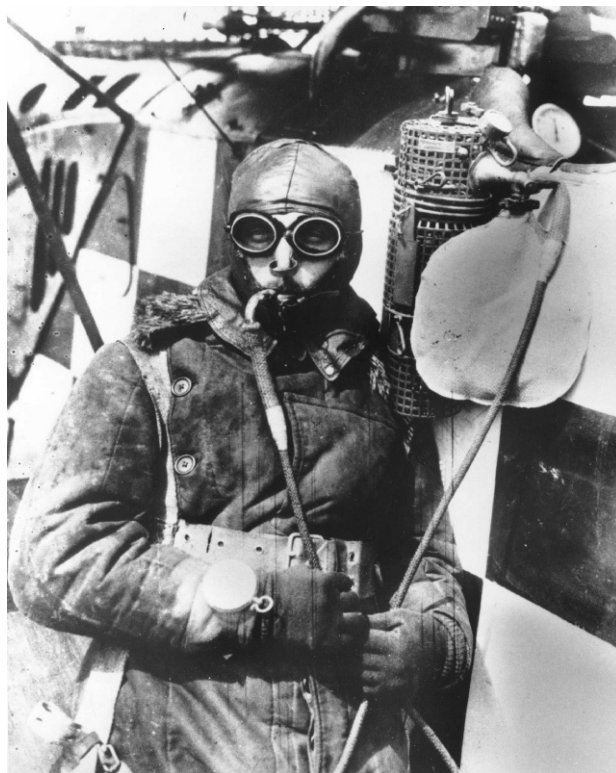
Figure 2.1. Circa 1918 German Imperial Flying Corp oxygen pipe system (courtesy Hamilton Sundstrand).
