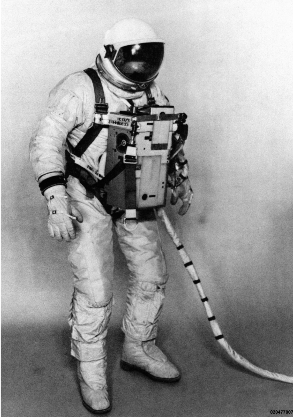
Figure A.5. Gemini V to XII DCC G4C suit and AiResearch ELSS (courtesy NASA).
