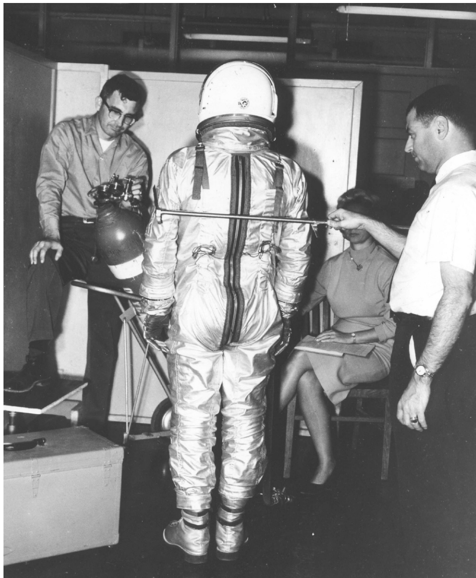
Figure 5.2.1. DCC Gemini rear-entry spacesuit (courtesy G. L. Harris).
