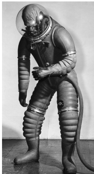
Figure 2.4. 1943 BFG XH-5 prototype suit (courtesy G. L. Harris).
