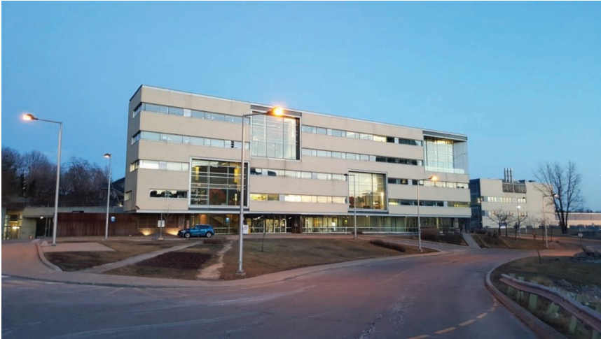
Figure 1.4 Photograph of the Bombardier research building where the interventional facility of the NanoRobotics Lab is located. The access to the car entrance to the underground level is on the left side of the photograph, while the interventional facility is located on the ground (main) floor on the right side of the photograph and at the far end of the building (in the back, not visible here).
