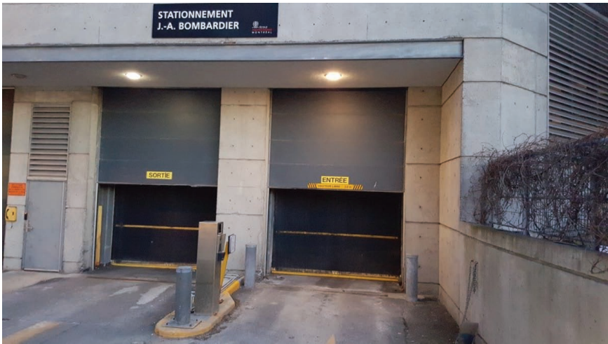
Figure 1.5 Photograph of the doors for the car entrances and exits to and from the underground level.
