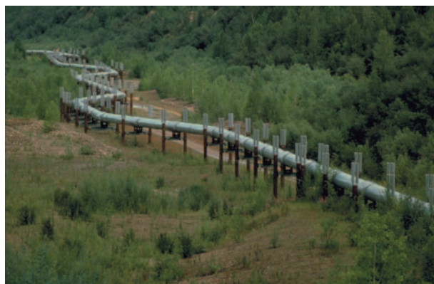
The 799–mi (1,286-km) long Trans-Alaska Pipeline is capable of transporting over 1.2 million barrels of oil per day.
