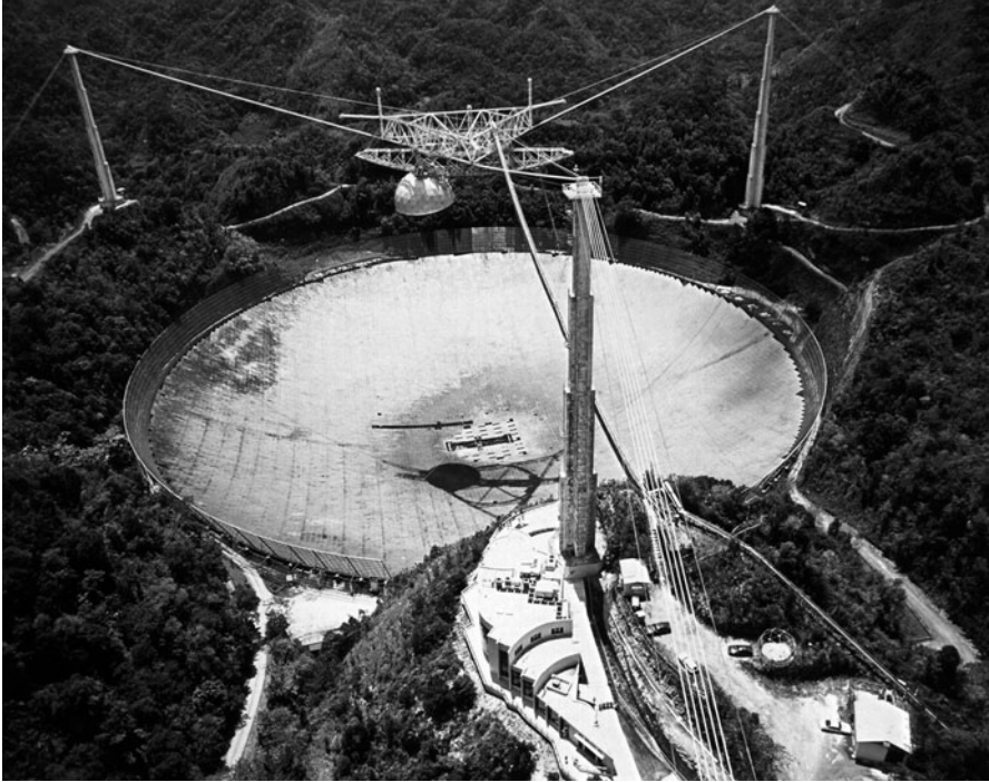
Fig. 4.13 Since its construction in the early 1960s, in a karst sinkhole in Puerto Rico, the Arecibo Observatory has been home to the world's largest single-dish telescope: the dish is 305 m in diameter, 51 m deep, and covers an area of about 8 hectares. The Chinese Five-hundred-meter Aperture Spherical Telescope will eventually outperform Arecibo, but the Puerto Rican telescope remains a formidable instrument. In principle, it could detect an alien transmission from the other side of the Galaxy. (Credit: H. Schweiker/WIYN and NOAO/AURA/NSF)
