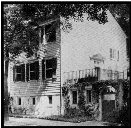
Volta Place after remodeling
