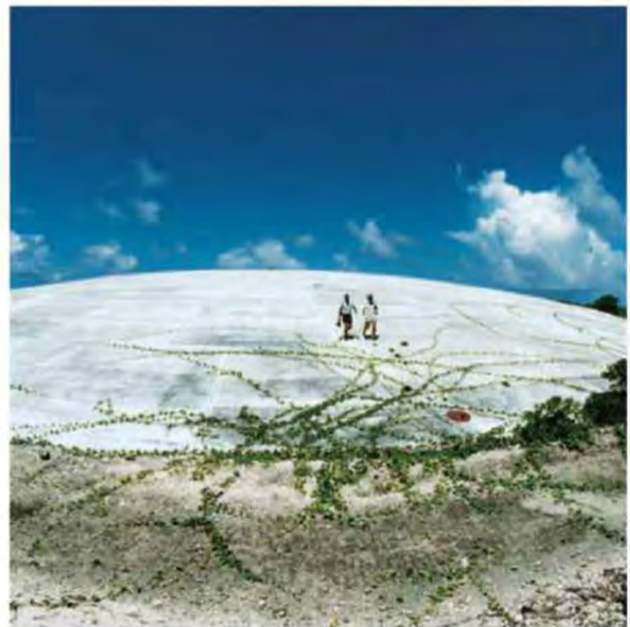
A CONCRETE DOME on Runit, one of the Marshall Islands, covers soil made radioactive by nuclear tests conducted by the United States in the 1940s and 1950s.
