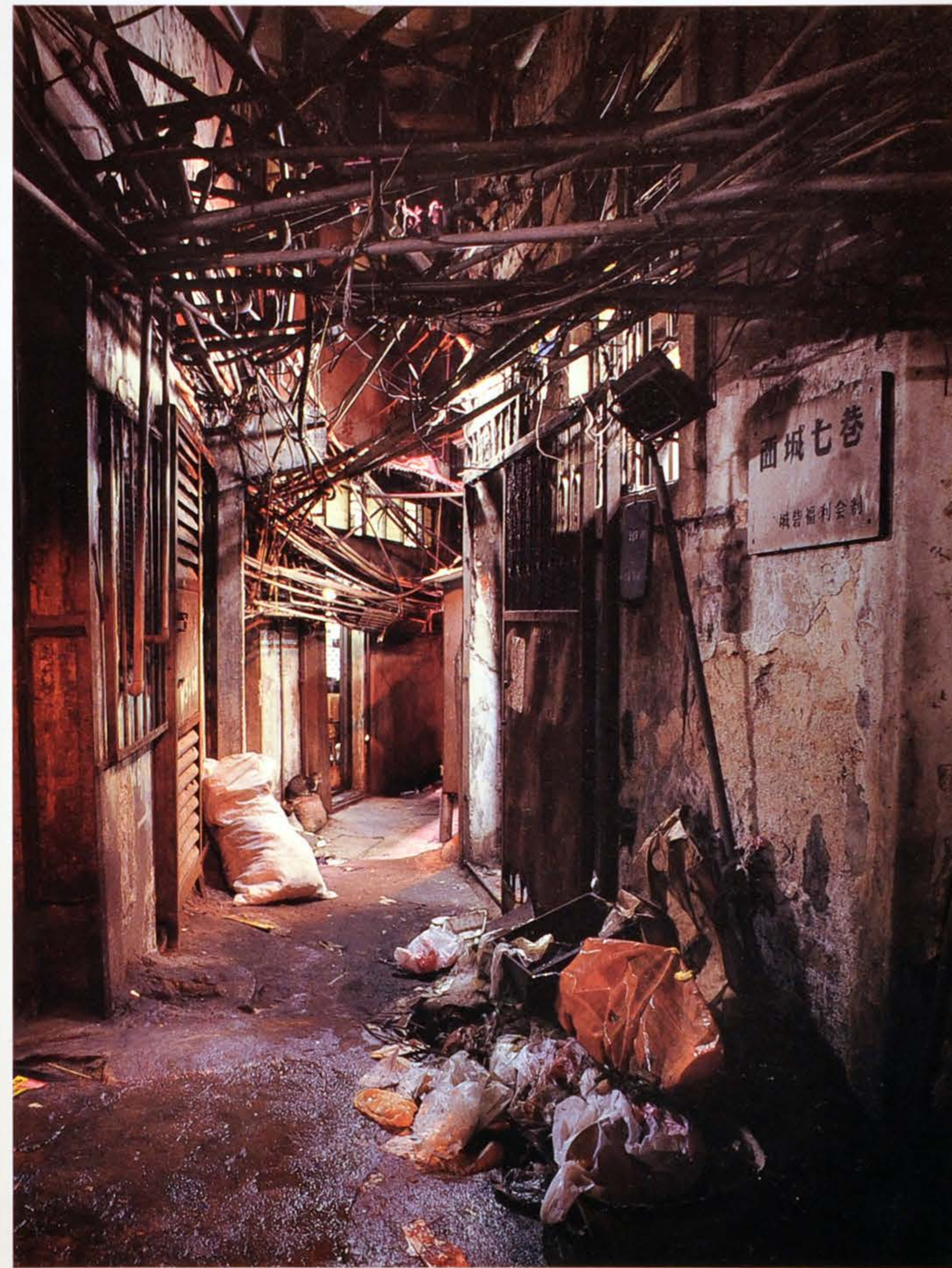
The visual chaos of piping — usually leaking, corroded and ingeniously patched up — channelled well water overhead. Buildings were rarely supplied with fresh-water or drainage connections, so all such piping had to be run externally. The residents' descriptions of well water varied by location: those in the northern sector complained that it was murky, heavy and malodorous, while others noticed a film of surface oil and black soot-like particles. What is certain is that, by the time of demolition, the over-exploited reservoirs beneath the City had become heavily polluted with urban and industrial effluence.
