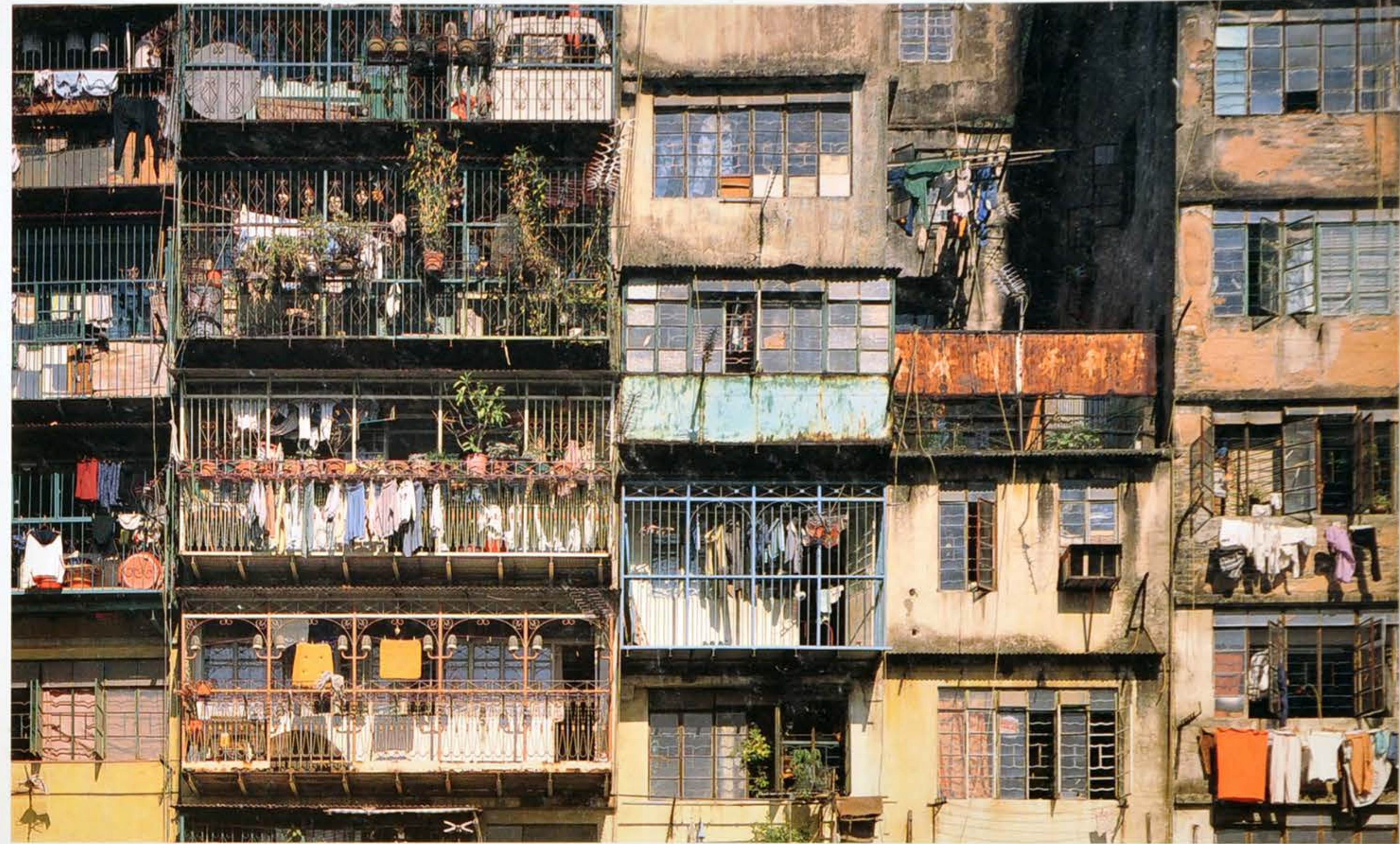
A typical section of external facade, horizontally uneven and animated with balcony life. Overleaf: In this photograph of 1990, the south side of the Walled City is seen facing on to the new public park, its formal greenery yet to take hold.
