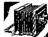
Camera with two tubes, for taking ster- eoscopic pictures. 525-WN
