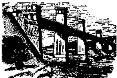
Tubular Bridge 3651R-M4
