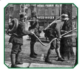
The WEX17 had a doughnut-shaped 2.9-gallon flame oil tank with a sphere inside the ring which held the nitrogen to discharge it. *Blauöl* ("blue oil"), the standard German fuel, also
