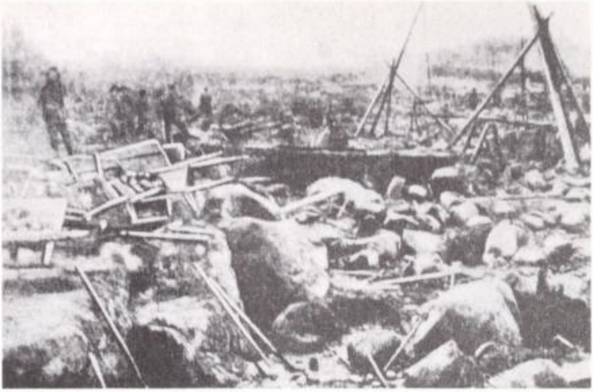
The wooden cranes
