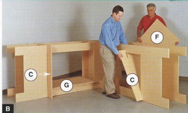
Interlock the slots in the ends (C) with the bases. Add the lower base shelves (F, G).
