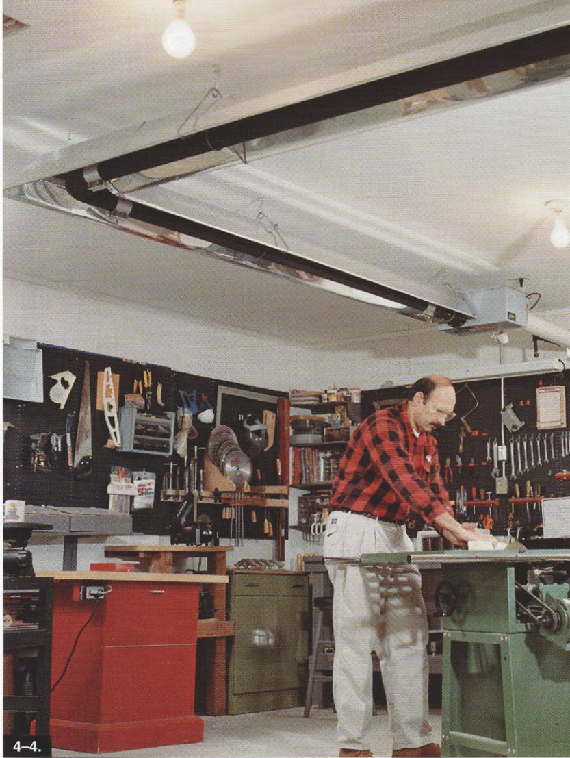
Radiant tube heaters, such as this one, are available in several sizes, and can be configured in straight, "U," and "L" shapes to fit the space.
