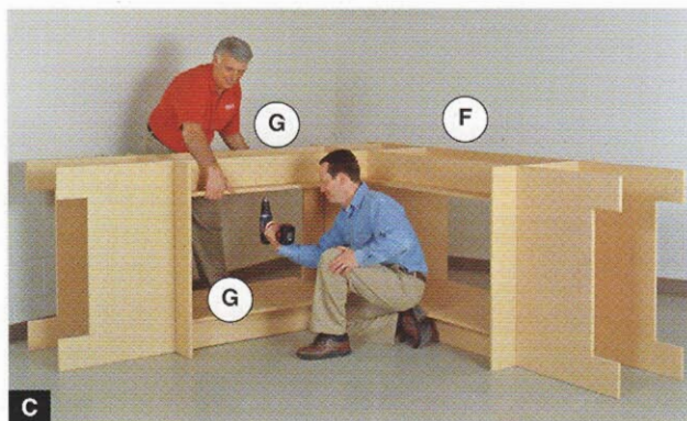
Drill pilot holes, and screw the upper base shelves (F, G) in place.
