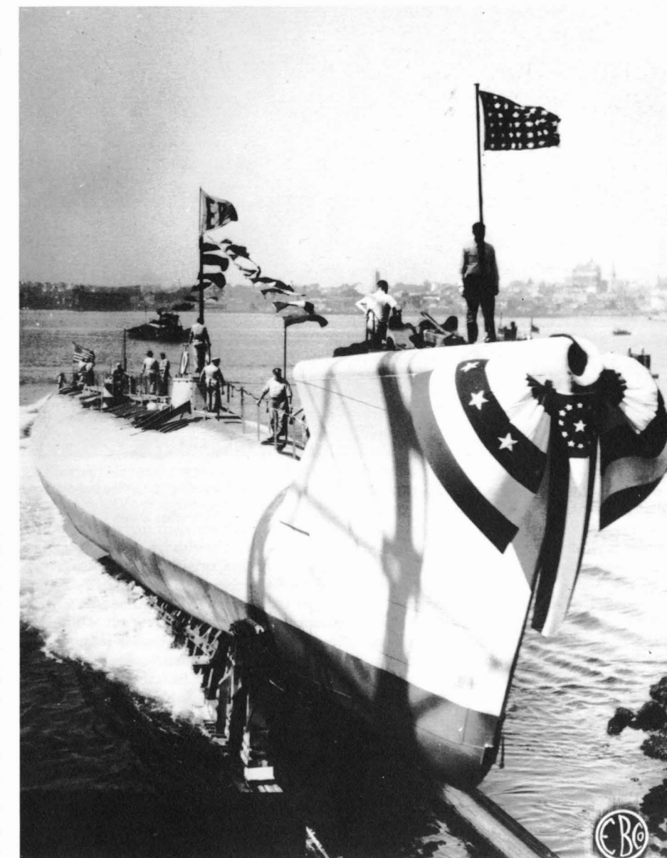
The incomplete US submarine Walrus (SS 437), being launched at Electric Boat on 20 September 1946, illustrates the tanking of a standard US fleet boat ( Tench class). She was complete except for her casing and her conning tower. The framing visible amidships belonged to the pressure hull, which was almost completely surrounded by tankage. The bow was complete because it contained the buoyancy tank. The Electric Boat house flag flies from the stub that would have led into the conning tower, which in American practice was (in effect) a secondary pressure hull. Walrus was delivered incomplete, and broken up in 1959.
