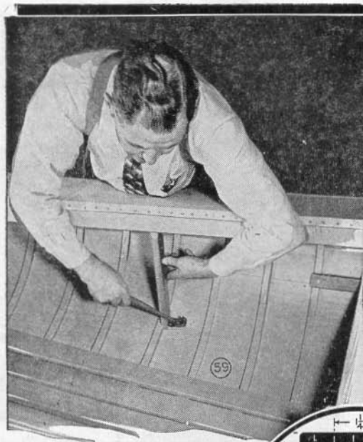
Braces along the sides of the cockpit carry the strain down to the ribs, thus giving ample strength to support persons sitting on the edge of the cockpit
