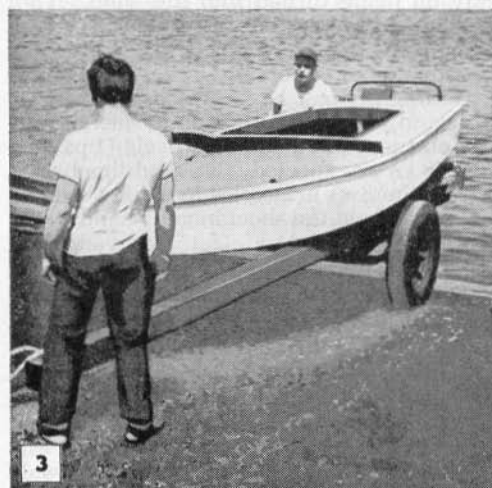
Below left, a beaching dolly is just the thing for launching small boats without the aid of a dock crane or where they are transported some distance for repairs. Right, approved manner of holding tiller and sheet
