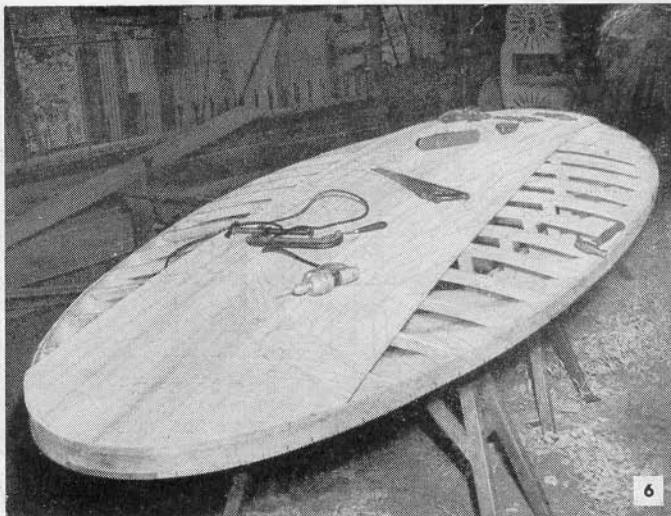
Original Scoot under construction. Note that the bottom planking is being applied after deck planking, a reverse procedure used by builder. It was found, however, more practical to plank the hull as described
