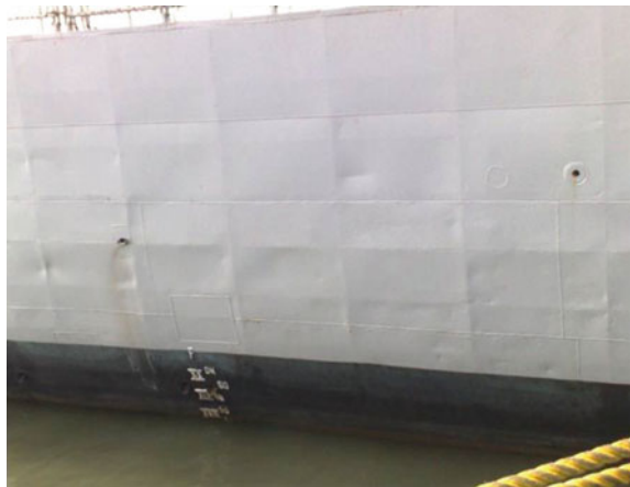
Fig. 17.1 Buckling of side shell panels
