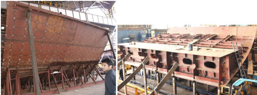
Fig. 5.4 Typical curved subassemblies
