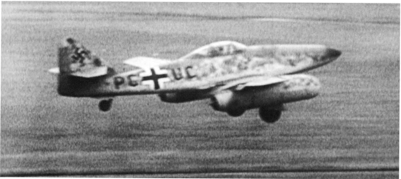
Fig 2.38 The first all-jet flight of the Messerschmitt Me 262 was with the V3 prototype (PC+UC) on 18 July 1942 at Leipheim when two Junkers 109-004 A-0 turbojets were used. The early Me 262 prototypes had tailwheel undercarriages, and the pilot, Fritz Wendel, had to tap the brakes at the right speed during take-off in order to lift the tail off the ground.
