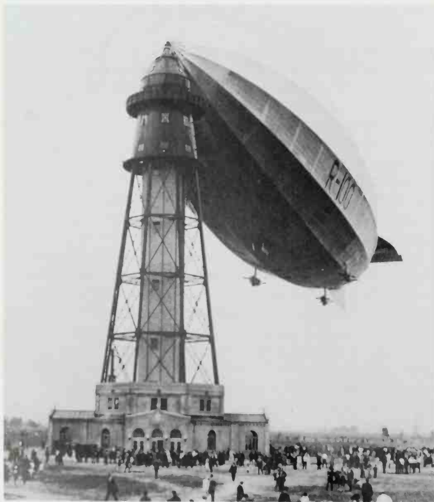
One million visitors from Canada and the United States came to look at the R 100 during its 13-day visit to Montreal in August 1930. Here, some of them cluster at the base of its 200-foot mooring mast or wait for an elevator ride up to the ship itself.
