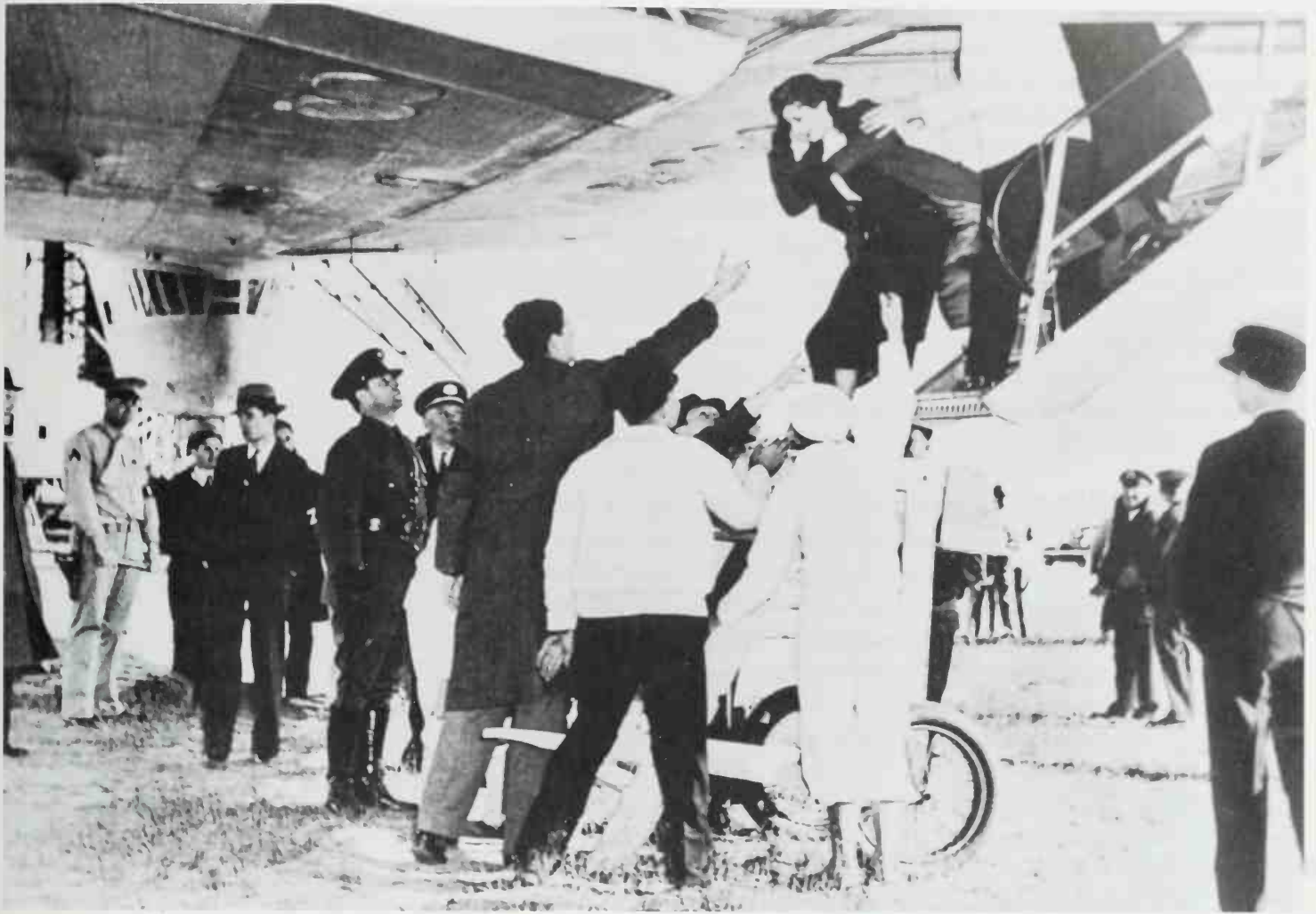
Passengers on the Hindenburg descend one of its gangways at Lakehurst after an Atlantic crossing in 1936. Bicycle-like wheels on a mobile landing stair allowed it to be repositioned as the wind moved the airship slowly at its mooring mast.
