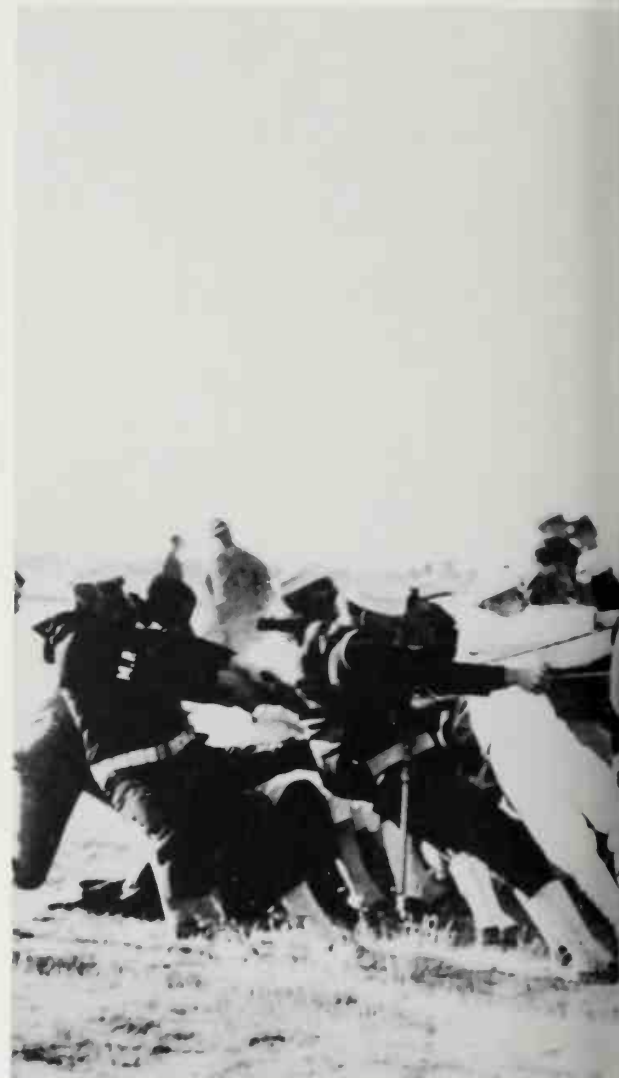
The ground crew at the Naval Air Station at Lakehurst, New Jersey, strains at the Hindenburg’s spider lines. While hovering to land, the buoyant ship was difficult to control in even a light breeze, and had to be hauled down manually for mooring.
