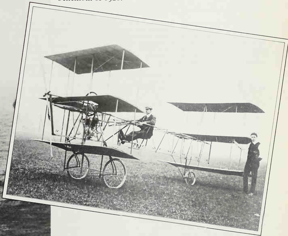
Above: Alliott Verdon Roe in his 1909 machine resorted not only to triplane wings but also a triple tailplane.
