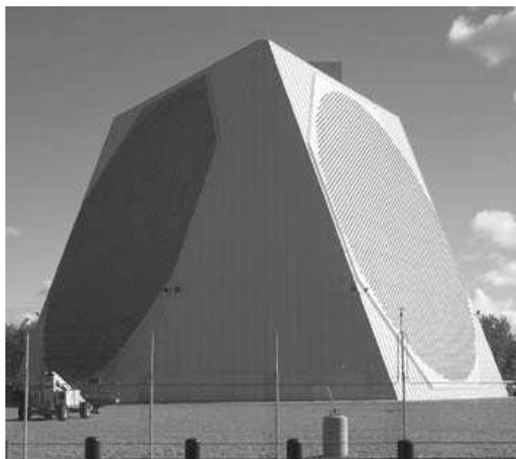
Figure 8.15. The PAVE PAWS antenna, part of the Ballistic Missile Early Warning System in Alaska (courtesy of U.S. Department of Defense).
