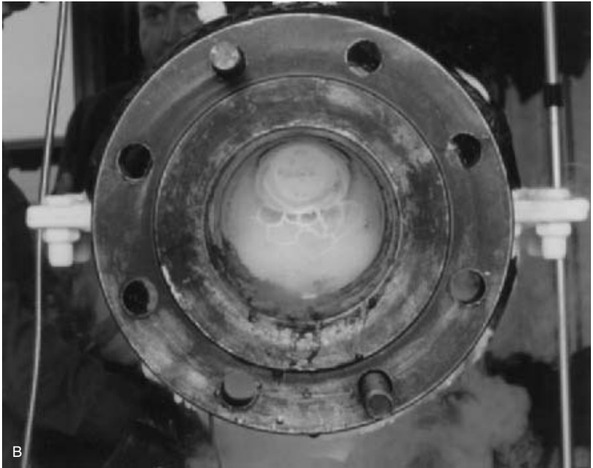
FIGURE B14.9b End view in which actual freeze plug can be seen. ( Team, Inc., Alvin, TX )
