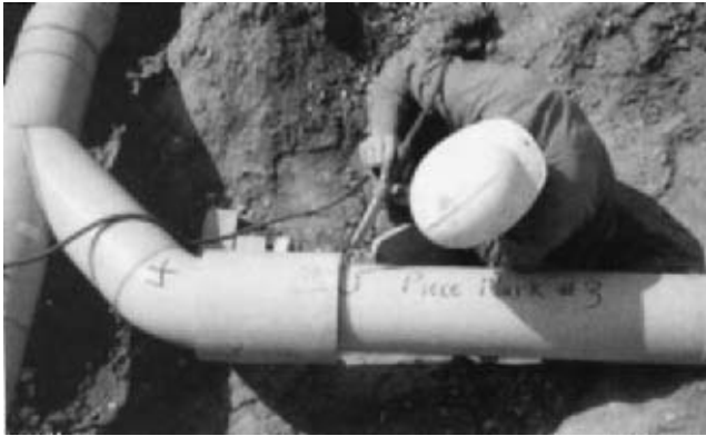
FIGURE B13.83 A tubular slip-coupling is bonded to the secondary containment coupling using hot-air welding in a thermoplastic double containment piping system. ( Grewe Plastics )
