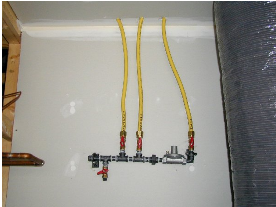
CCST yellow gas pipe to a pressure regulator with a three-piece ground joint. Some plumbing codes will call this joint a Left & Right Nipple. Any joint coupling is required to be in an accessible area.
