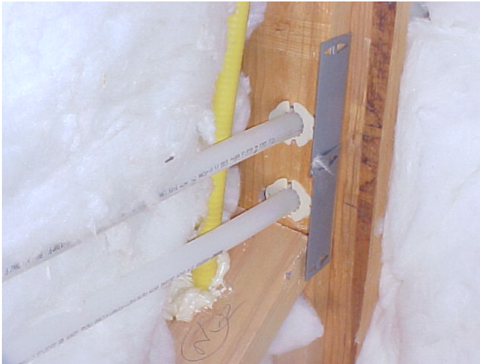
Combination waste and Vent system, Island Sink set-up 2 inch minimum vent The Foot Vent will go up the adjacent wall. Below, nail plate protection is necessary even for copper lines.
