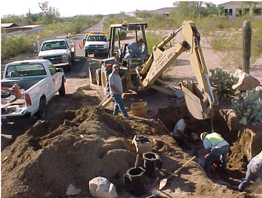
Repair crew replacing three tapping valves that blew out during a leak.
