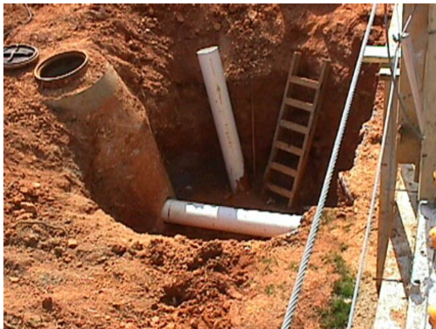
Sewer lateral going into a manhole.
