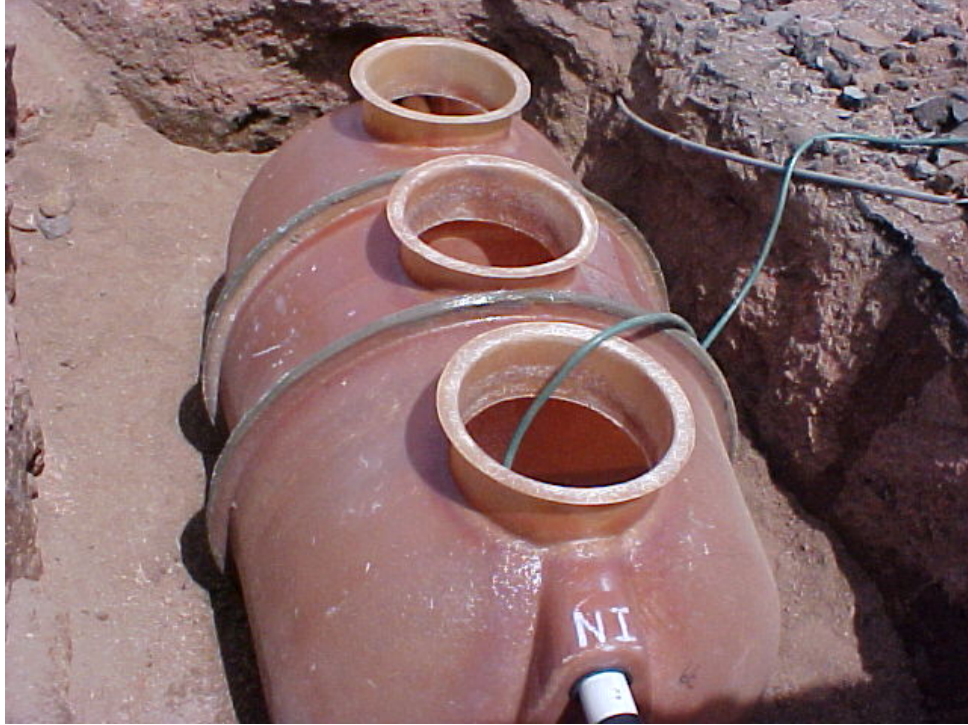
Three Compartment Grease Interceptor
