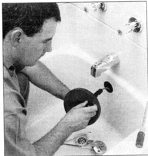
Clogs of hair are often found wrapped around the pop-up drain assembly.
