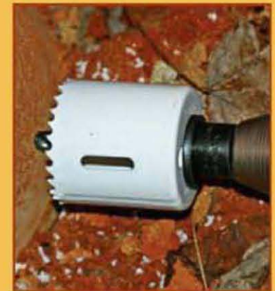
29 | Drilling the Well Casing
