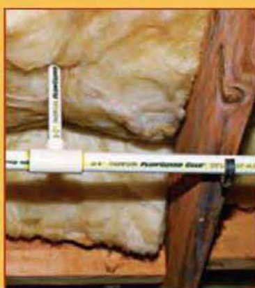
175 | Running the Lines
