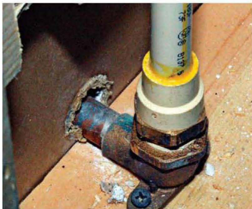
A drop-ear elbow with female threads can terminate nonmetal pipe in the wall, with copper extending through the wall for the fixture.
