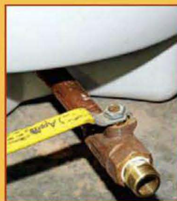
129 | Installing Full-Flow Drains
