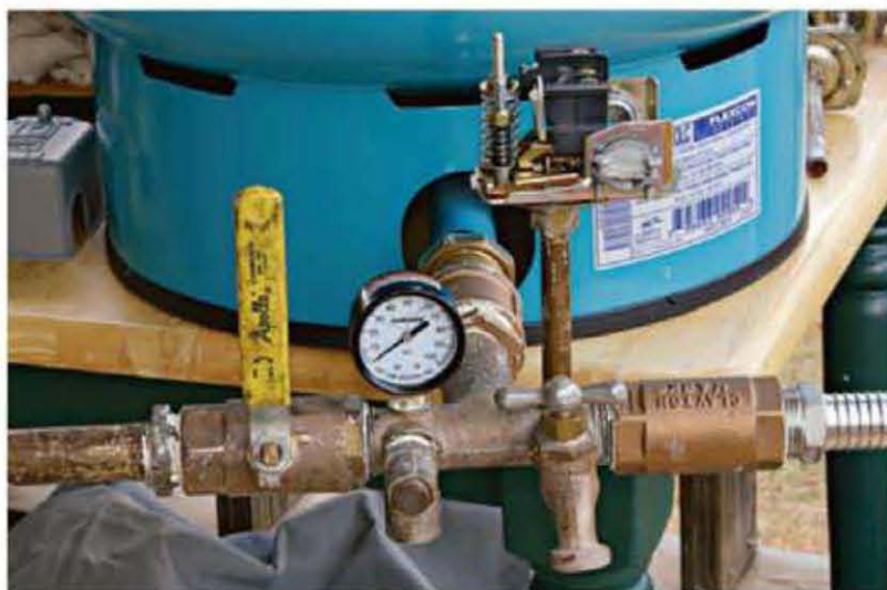
The purpose of a tank T is to have one place to attach the many different fittings and control items needed at the tank.
