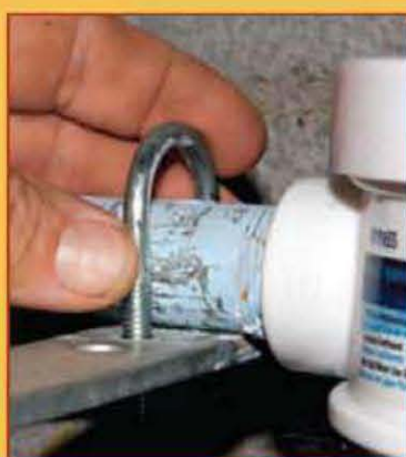
70 | Replacing and Securing a Filter
