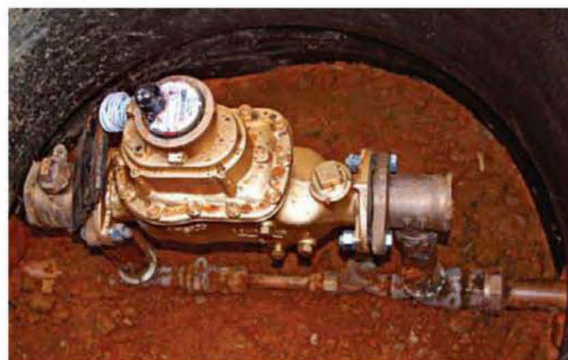
Larger or deeper water meters require an inverted plastic culvert as a box.
