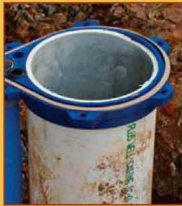
32 | Installing a Watertight Well Cap
