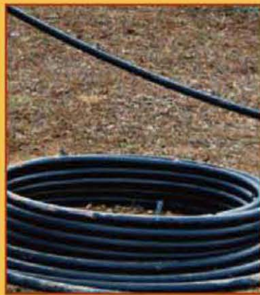
35 | Prepping the Pipe
