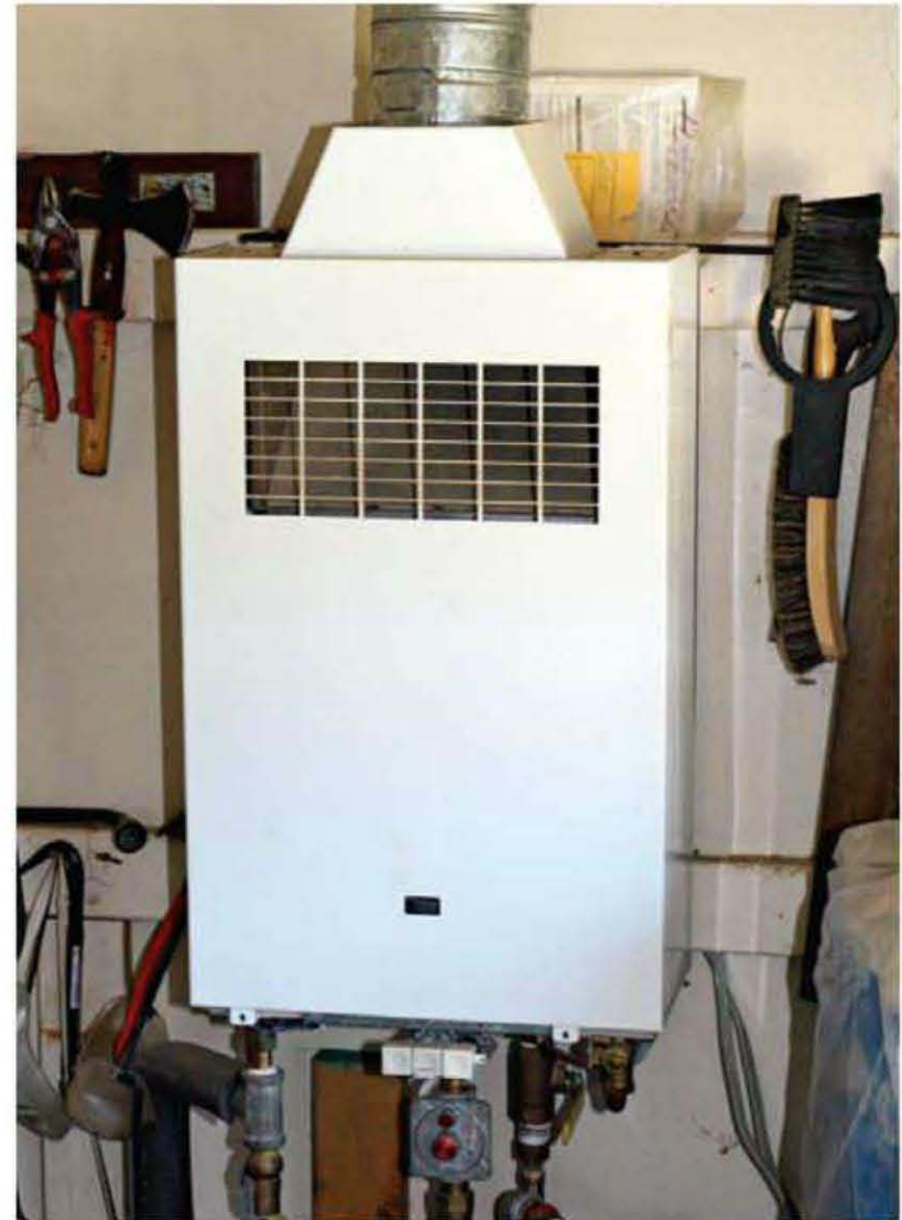
Demand heaters heat water only when it's needed, but they have a host of problems.
