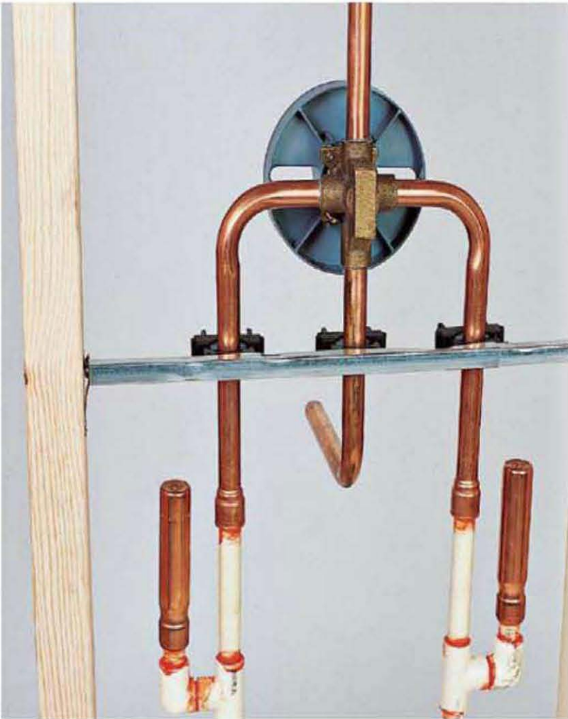
The water lines to a shower, tub, or tub shower, as well as the valve itself, can be mounted to a simple metal-bracket. (Photo courtesy Sioux Chief Manufacturing.)
