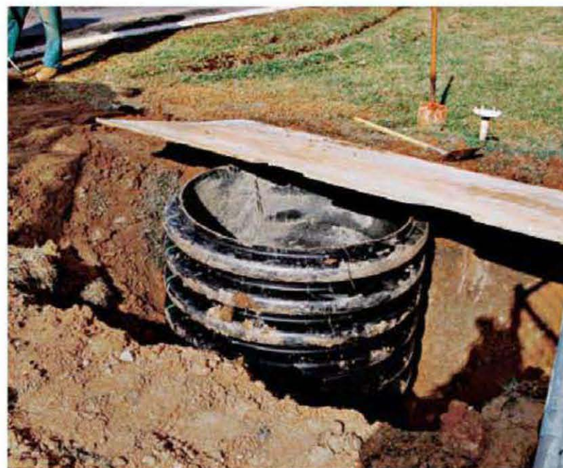
Larger or deeper water meters require an inverted plastic culvert as a box.
