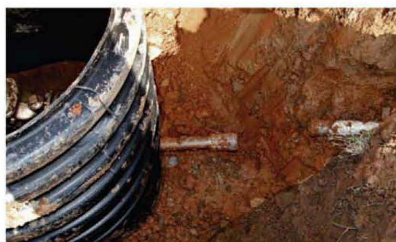
Larger water meters , like this 2-in. unit ( top ), come with built-in backflow and water pressure devices and a bypass below the meter. A unit this size will supply a very large house. It comes with about 3 ft. of 2-in. copper pipe extending from the meter box ( bottom ) so the plumber can tie into the water meter line without having to get inside the meter box. Here 2-in. polyvinyl chloride (PVC) is used.
