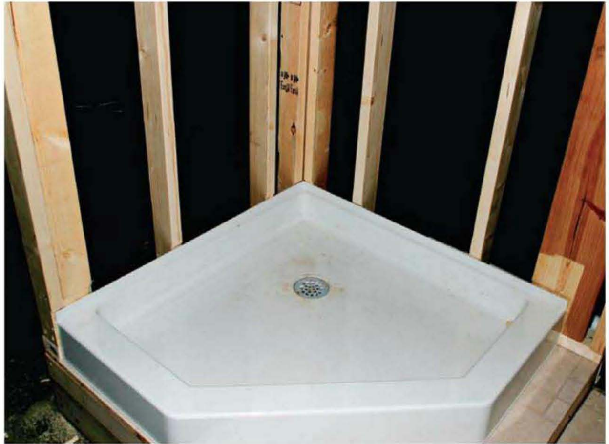
The wall on the left has a stud dead center that would block the installation of a spigot. The wall on the right is open in the middle—its stud is not in the way. When studs are in the way, cut their support nails with a recip saw and move them to the side.
