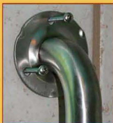
207 | Installing a Grab Bar
