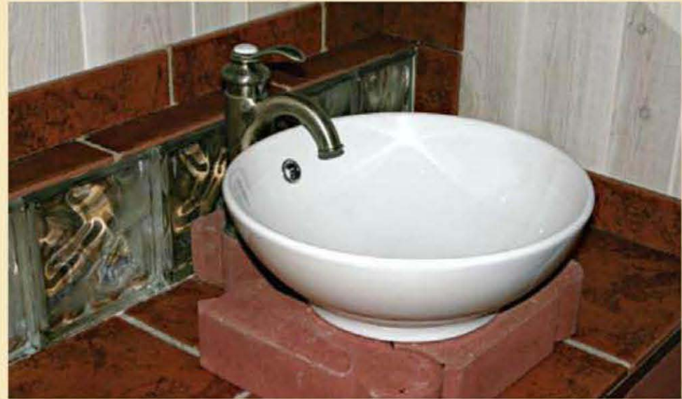
Ceramic vessel sinks (above) look great. Sinks with overflows have hollow channels (left). Allow for them when cutting out lav tops.
