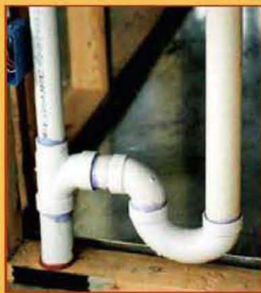
158 | Running the Lines
