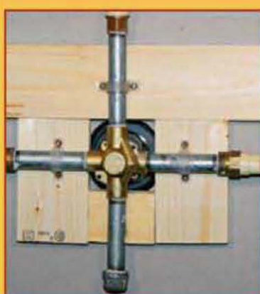
182 | Showers, Washers, and Refrigerators
