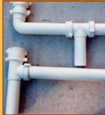
187 | Installing Kitchen Drains
