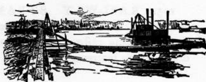
1259. MARINE DREDGE, discharging on the shore through a long floating pipe. Pipe buoyed by pontoons. For harbor work.
