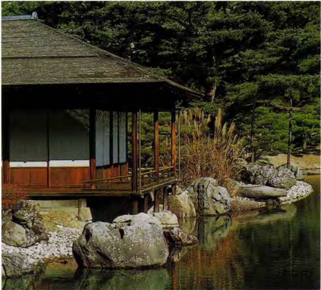
Rock foundations for the stilts supporting Kikugetsu-tei Pavilion in Ritsurin Park, Takamatsu.
