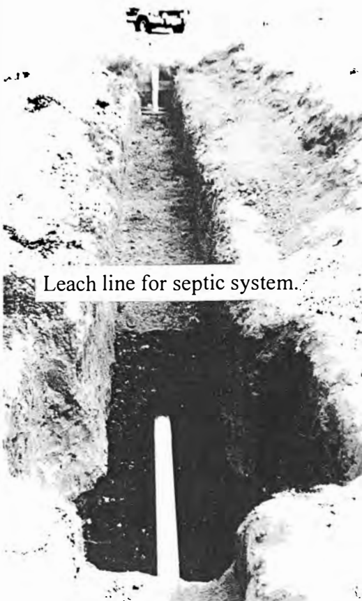
Installing the leach line.
