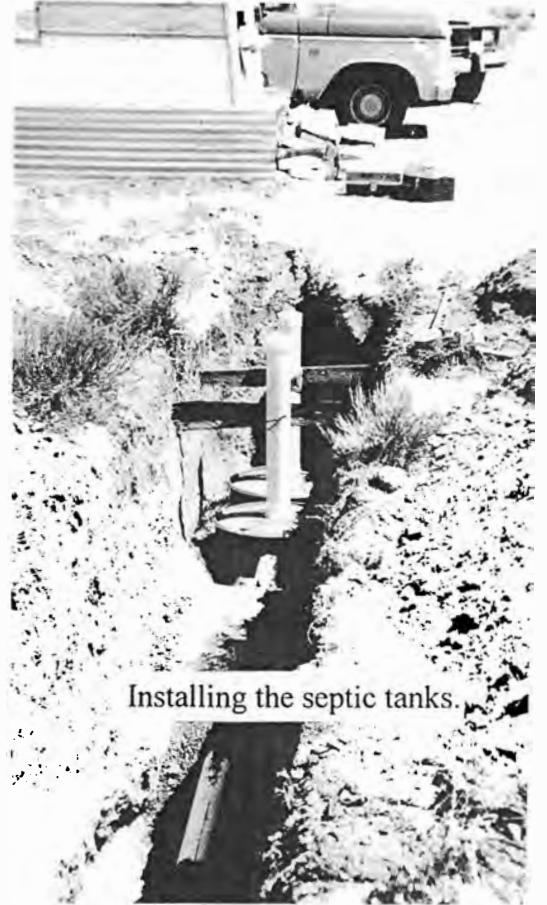
Septic barrels when first placed in holes.
