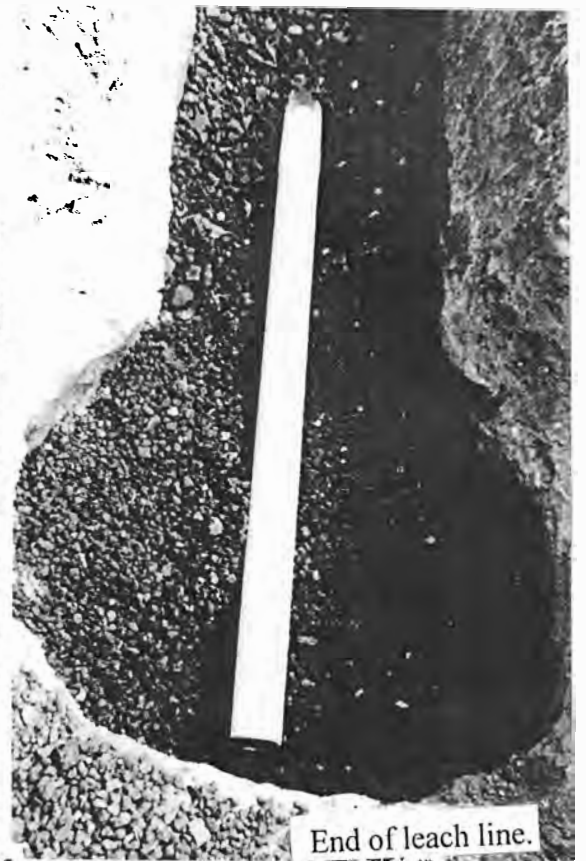
Installing the leach line.
