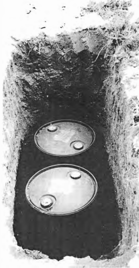
Septic barrels when first placed in holes.
