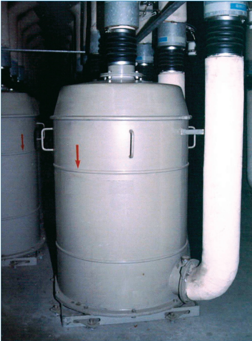
Figure 3-4 A canister-type filter unit is often used for Class 1 Safe Rooms to maximize storage life of the filters. SOURCE: BATTELLE
