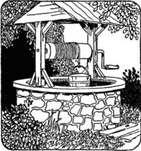
Dug stone well, with cover and windlass to lift water bucket
