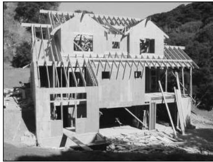
Figure 1-1: A house in progressive stages of construction. From site prep through foundation, framing, and exterior work, this home took more than eight months to build.
