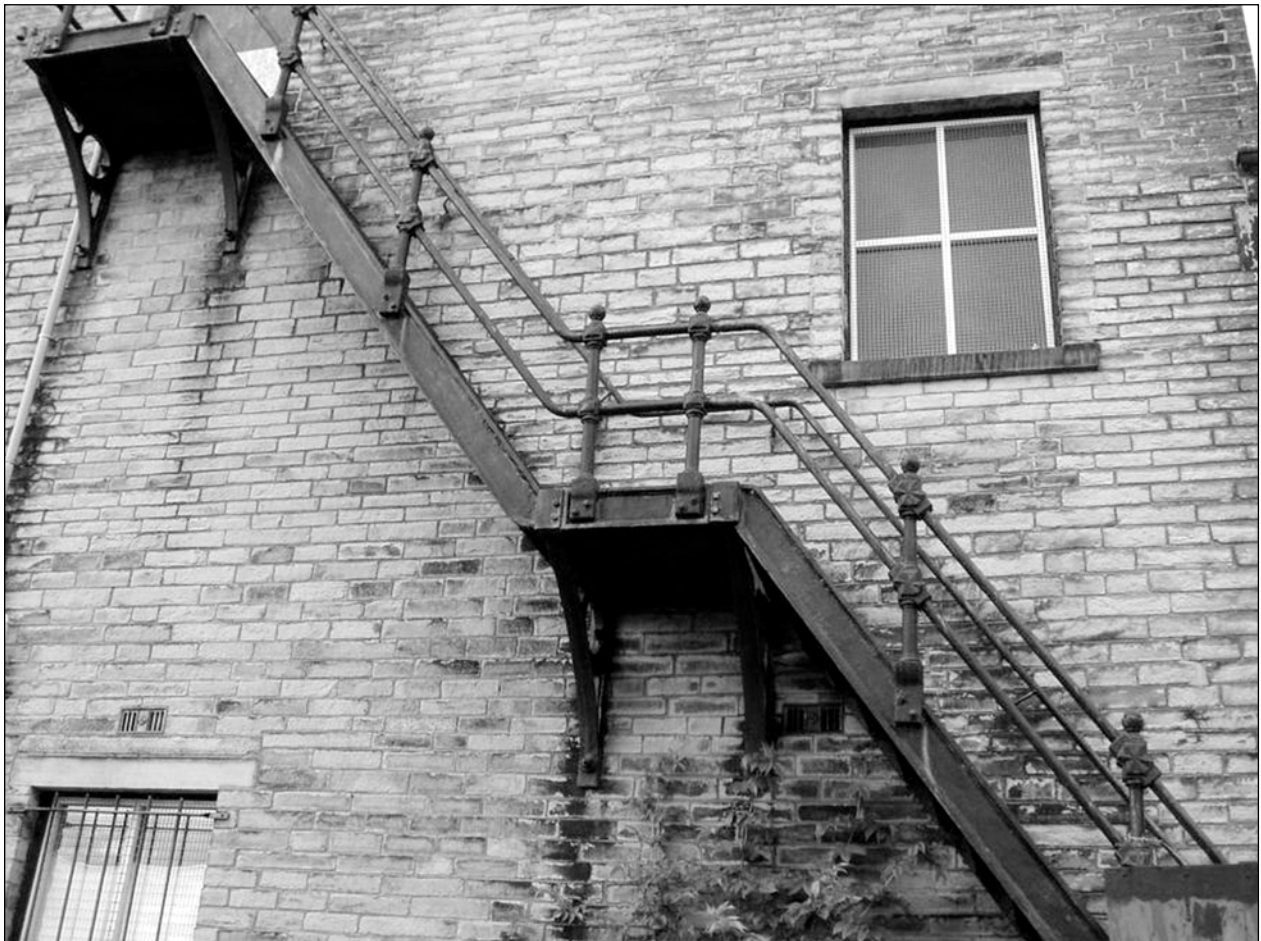
Figure 7.3 Cast-iron staircase immediately prior to reclamation and reuse
