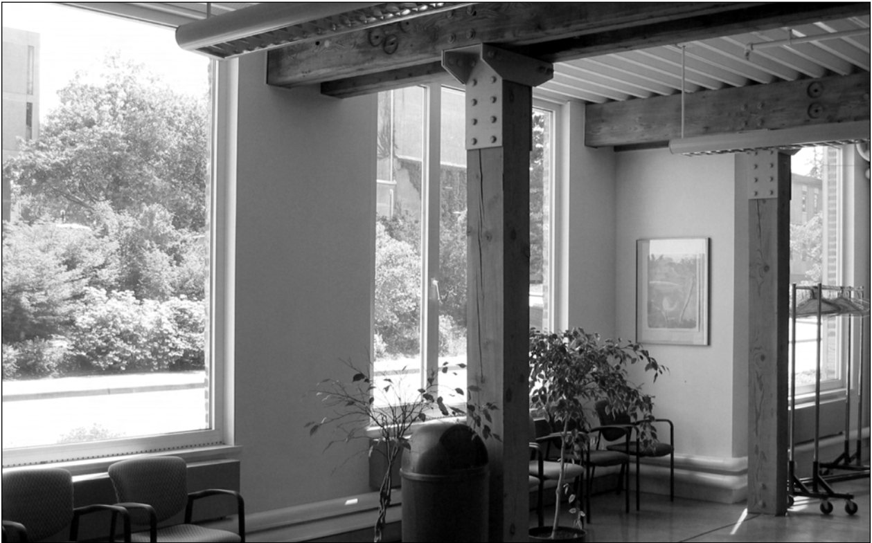
Figure 2.4 Choi building: Reclaimed structural timber
