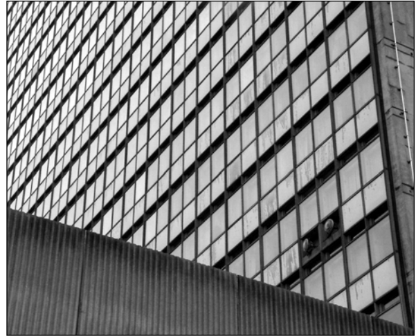
Figure 6.5 Piccadilly Plaza, Manchester, UK: The curtain wall prior to refurbishment
