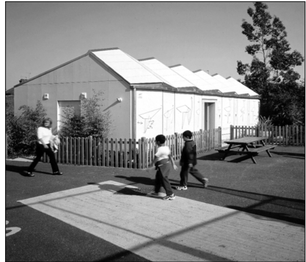
Figure 2.11 New classroom at Westborough School, constructed largely from cardboard made from recycled paper
