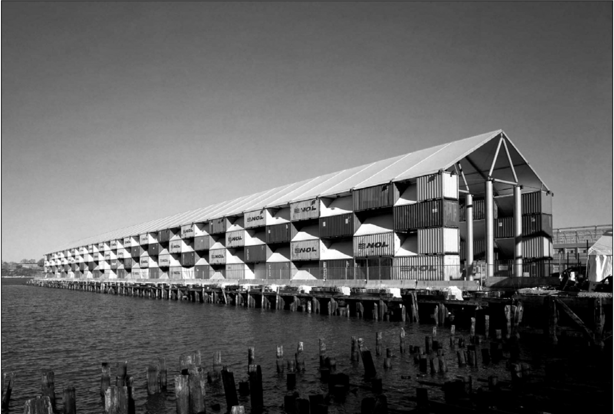
The Nomadic Museum, New York City, 2005 – Architects: Shigeru Ban and Dean Maltz; engineers: Buro Happold
