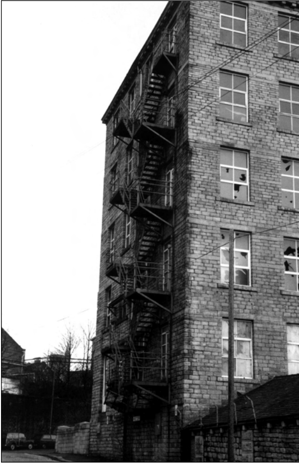
Figure 5.7 Load-bearing stone walls at the East Mill, Huddersfield before refurbishment
