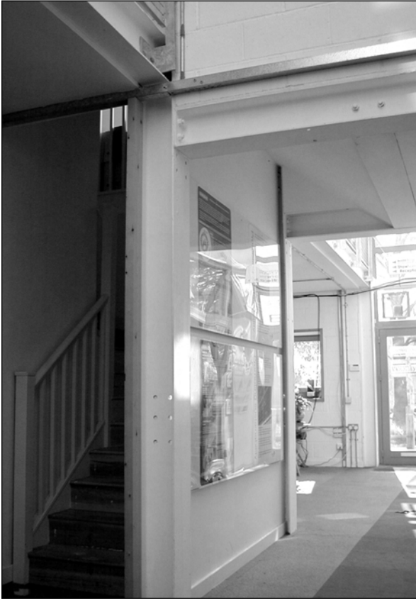
Figure 2.2 Reclaimed steel columns and beams at BedZED
