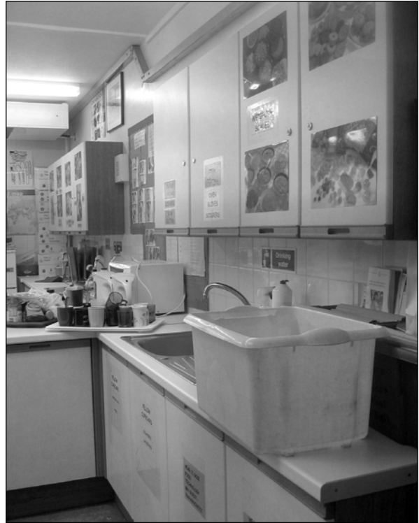
Figure 2.9 Cupboards will be reclaimed from school to be demolished
