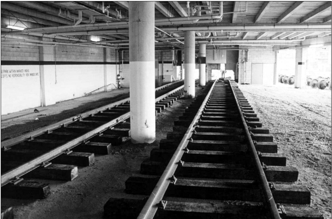
Figure 5.4 Rail tracks installed at ground level
