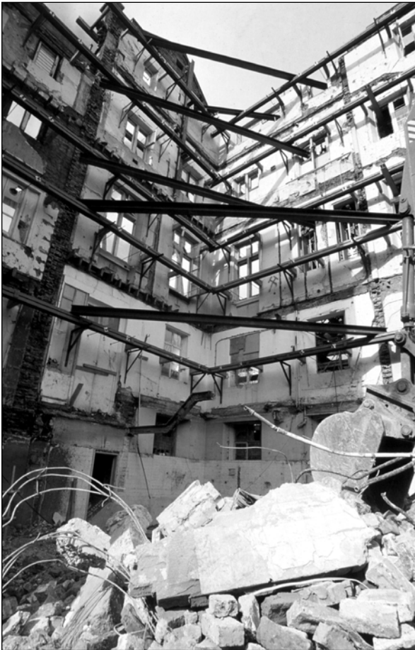
Figure 6.2 The retention structure for Shorts Gardens façade
