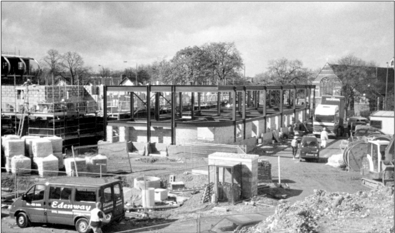
Figure 2.19 Structure of new building constructed with reclaimed steel
