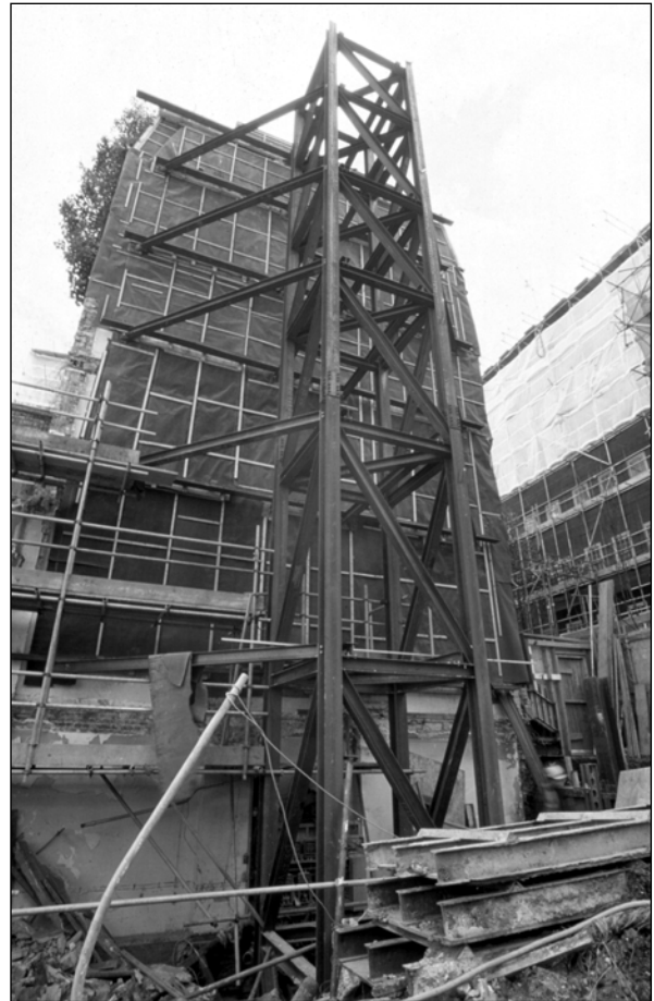
Figure 6.3 The retention structure for the Georgian terrace façade
