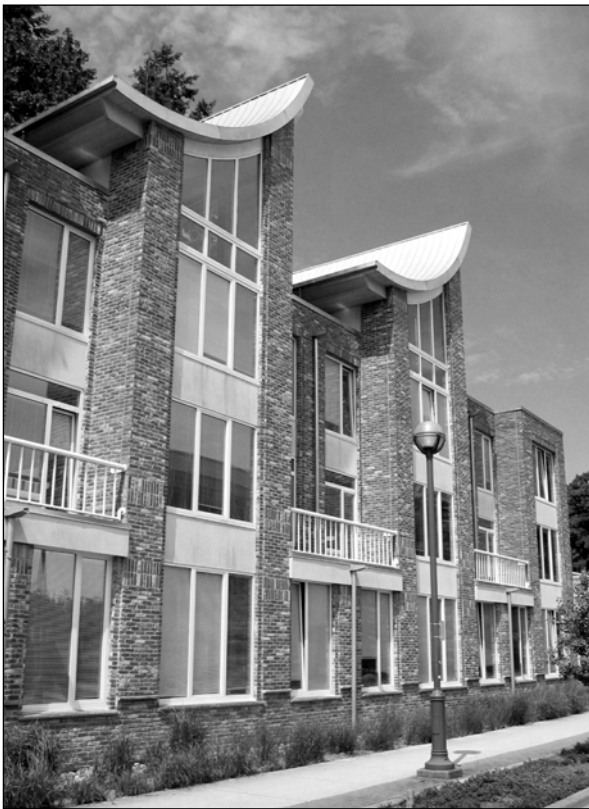
Figure 2.3 Choi building: Exterior, showing reclaimed brickwork
