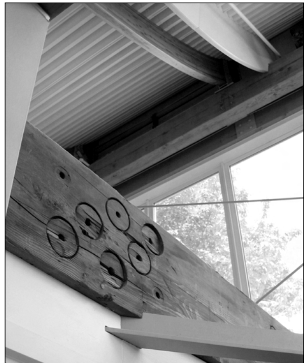
Figure 2.5 Choi building: Detail of structural timber showing evidence of its previous life
