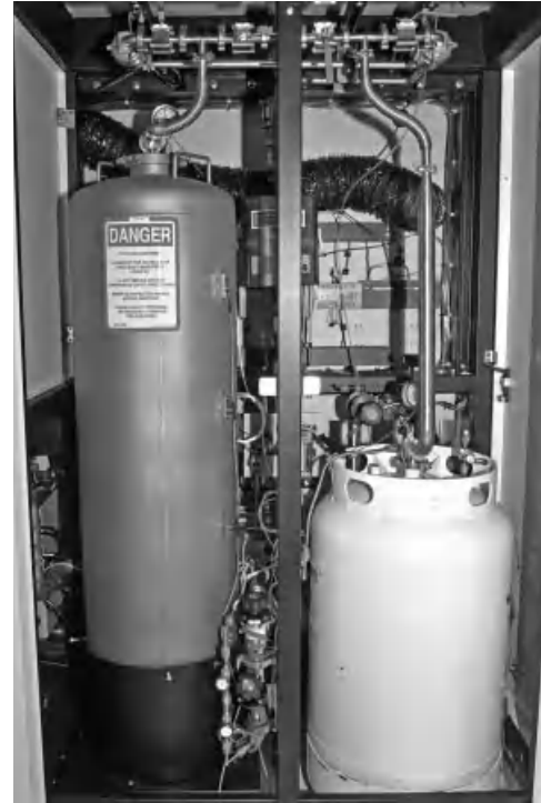
FIGURE 23-11. View of emergency purge air-cleaning system for a single toxic gas cylinder.
