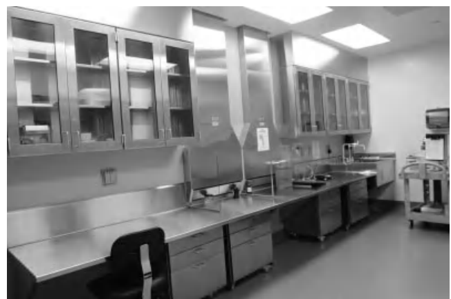
FIGURE 22-5. View of slot exhaust dissection stations in necropsy laboratory.
