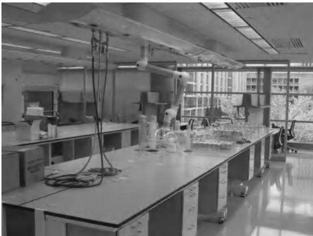
FIGURE 2-8B. View of an overhead utility carrier. (Courtesy: Massachusetts Institute of Technology, Cambridge, MA)
