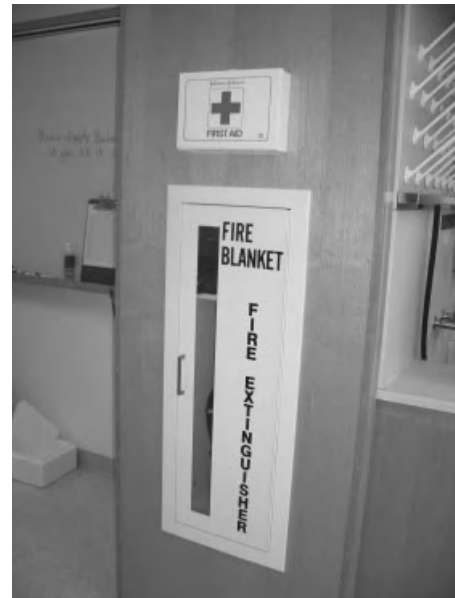
FIGURE 2-11D. View of laboratory entry with first aid kit, fire blanket, and extinguisher. (Courtesy: Washington University, St. Louis, MO)
