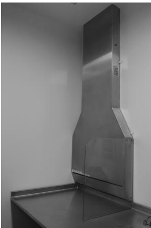
FIGURE 32-8. View of a slot hood in a pathology laboratory.
