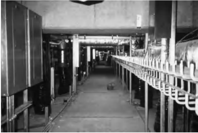
FIGURE 1-19A. View of interstitial floor at Fredrick Hutchinson Cancer Center Research Laboratory.
