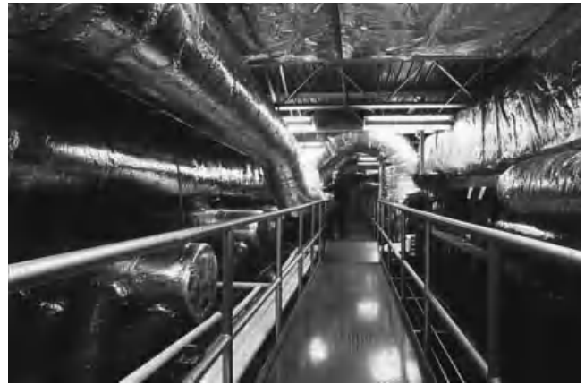
FIGURE 1-20A. View of interstitial space at Bausch and Lomb research building.
