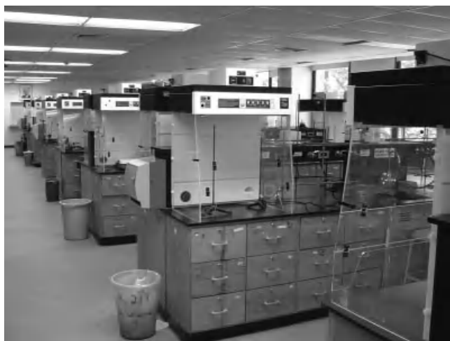
FIGURE 32-11. View of a ductless fume hood in a teaching laboratory. (Courtesy of Erlab Inc., Rowley, MA.)
