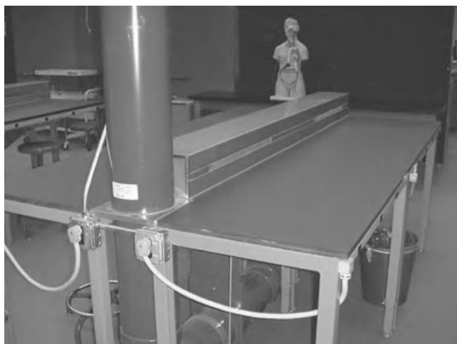
FIGURE 16-5. View of slot exhaust device at teaching laboratory benches.
