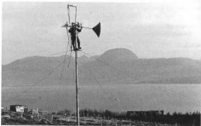
Fiting a windmill rotor at the top tower using pulleys.
