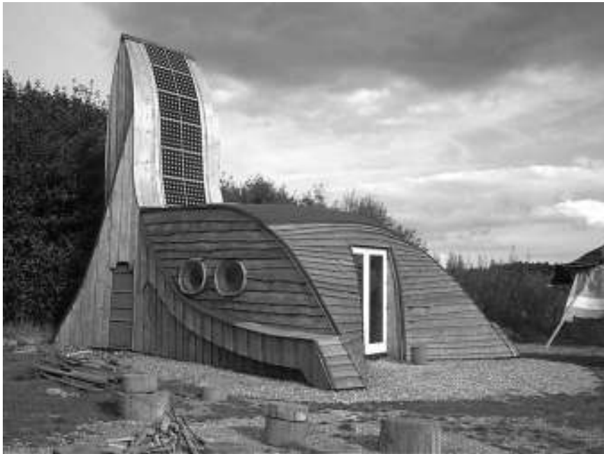
Figure 10-38 Photovoltaic cells creatively integrated into a building fabric. Image courtesy Jason Hawkes.
