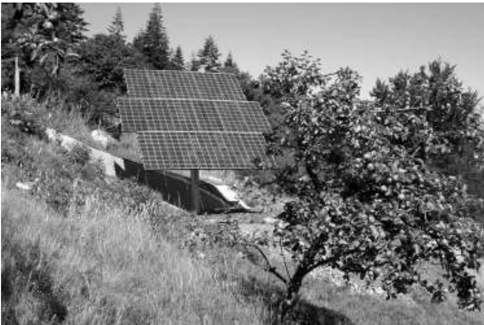
Figure 14-1 Solar tracker at Llanrwst, near Snowdonia, Wales. Image courtesy Dulas Ltd.
