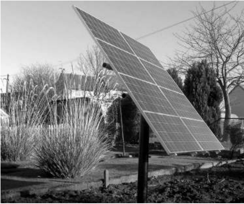
Figure 14-5 Solar tracker on the property of Mr Howie, Scotland. Image courtesy Dulas Ltd.
