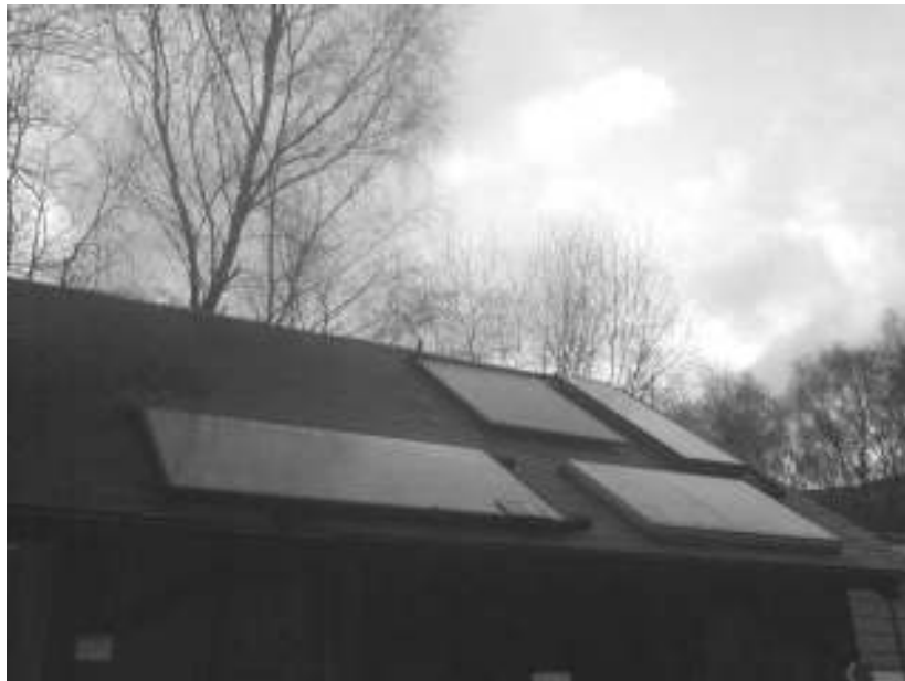
Figure 4-5 An array of different solar thermal cells on a roof.
