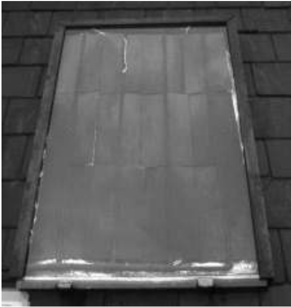
Figure 4-7 A home-made clip fin collector.
