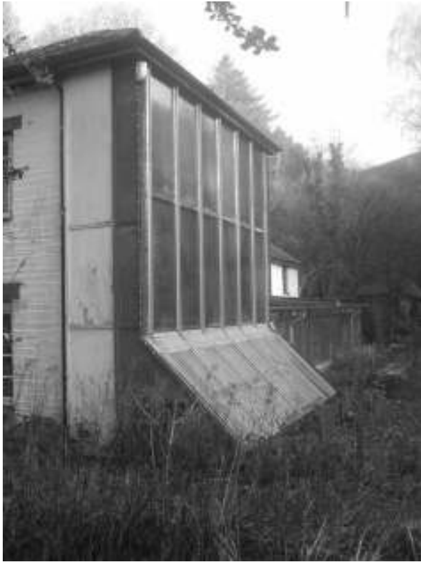
Figure 5-1 Trombe wall at CAT, U.K.
