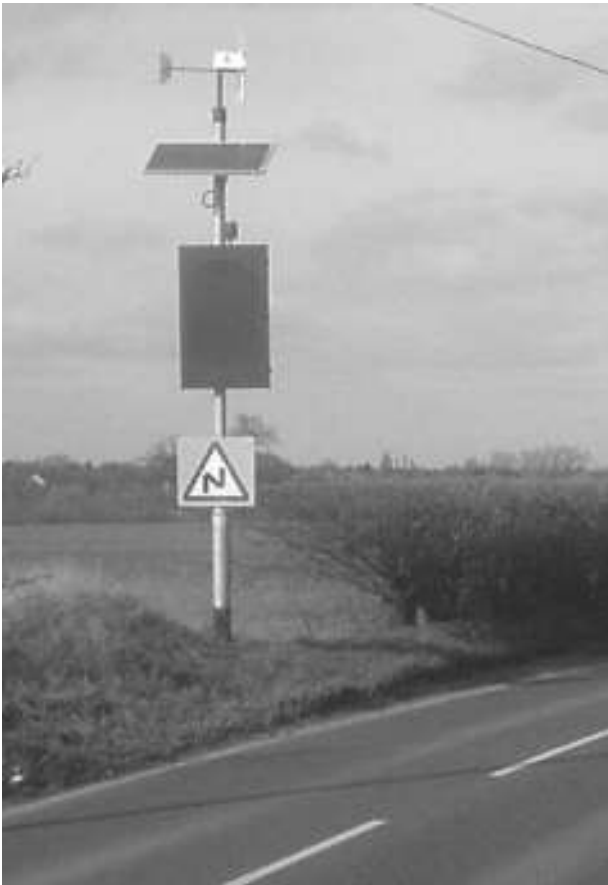
Figure 10-36 A road sign powered by renewable energy.
