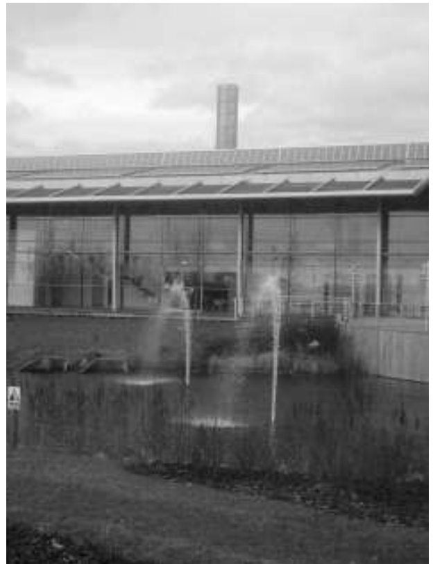
Figure 9-1 Photovoltaic-powered fountains enhance the CEME, U.K.
