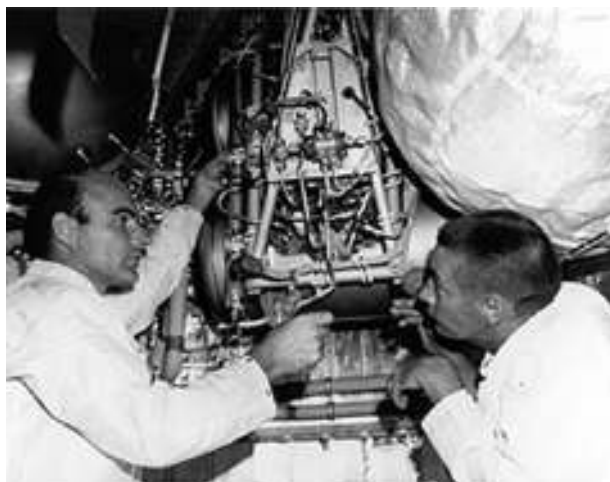
Figure 1-17 The alkaline “Bacon Cells” used in the Apollo missions. Image courtesy NASA.
