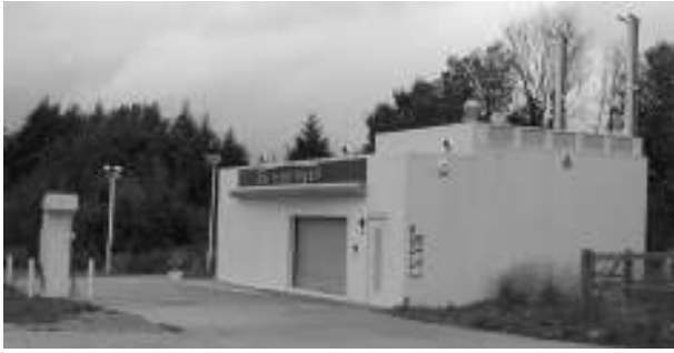
Figure 13-7 A specially constructed hydrogen filling station.
