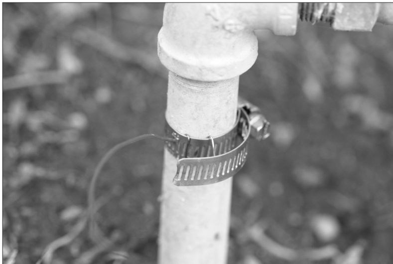
Figure 2-6: A good ground connection.
