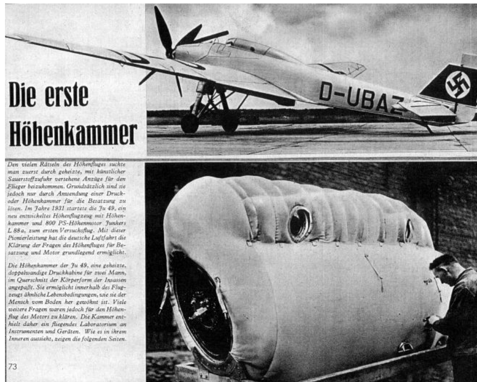
Figure 5.8: The Junkers Ju49, with coated pressure cabin. Taken from “ADAC-Motorwelt”, 1935.
