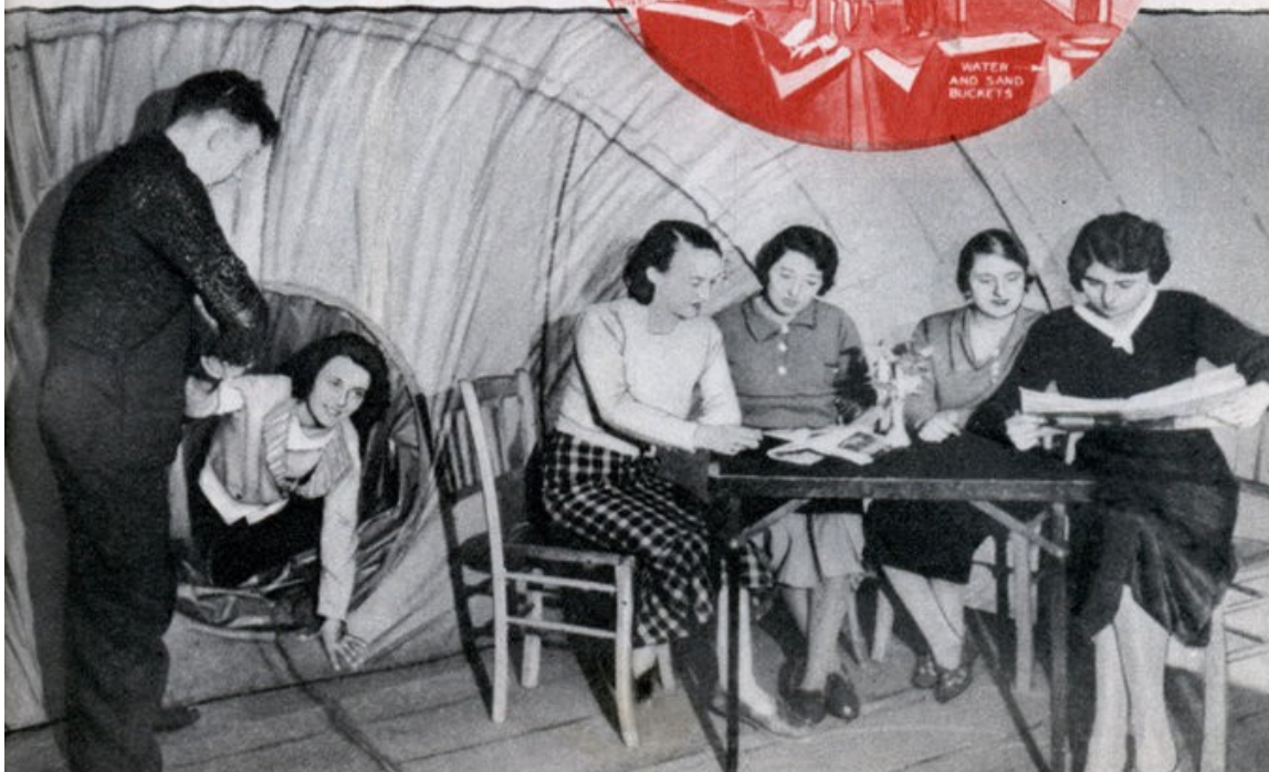
Circle—Interior of proposed shelter room showing supplies and arrangement to provide 12 hours protection without need of ventilation. Wet blankets guard the entrance to shelter rooms against penetration by fumes. Below—Woman entering an impermeable French "balloon" type gas shelter. Inflated by a pneumatic pump, it is quickly set up.
