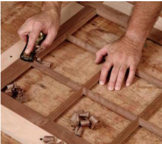
Plywood strips screwed to an assembly table hold this door for planing.
