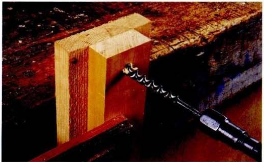
ABOVE: For maximum efficiency, the waste piece needs to run down to the floor.
