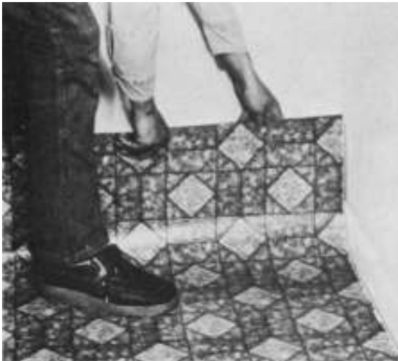
Figure 2-9 Resilient flooring is first laid in a room.
