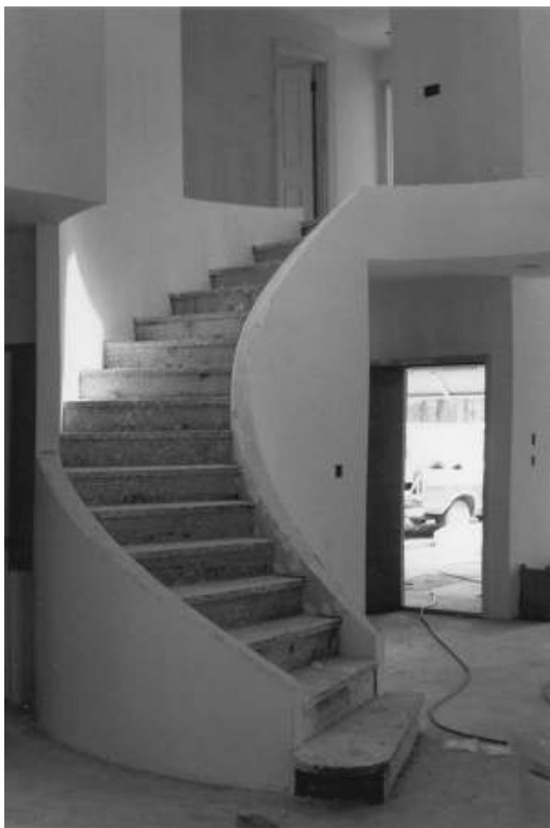
Figure I-22 Stairway enclosed with drywall and step at bottom being installed.
