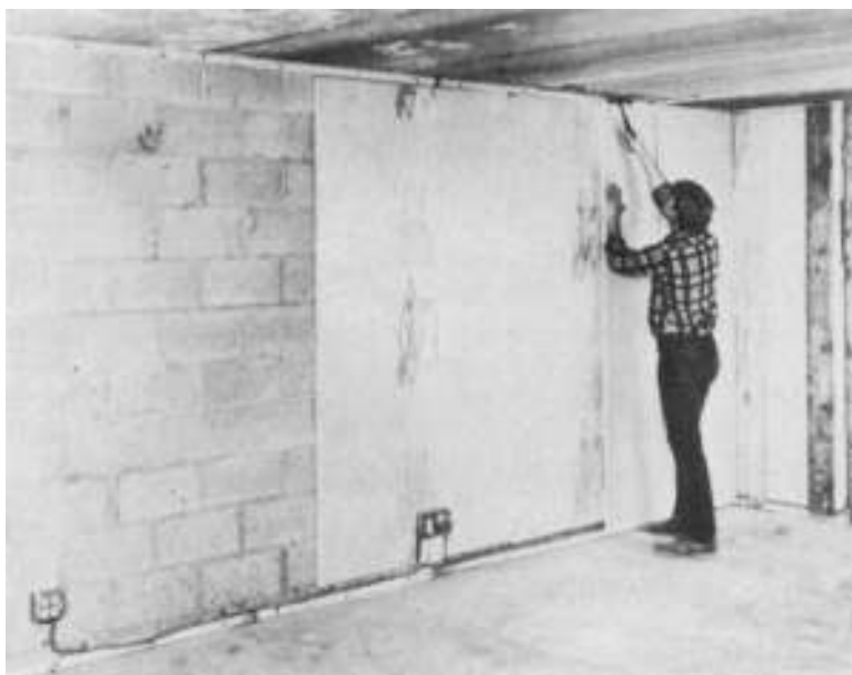
Figure 8-1 A block or masonry wall is a good candidate for Styrofoam or urethane board insulation. (Courtesy of Dow)
