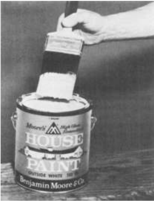
Figure 5-2 Brush should be loaded no more than two-thirds when painting. (Courtesy of Benjamin Moore)
