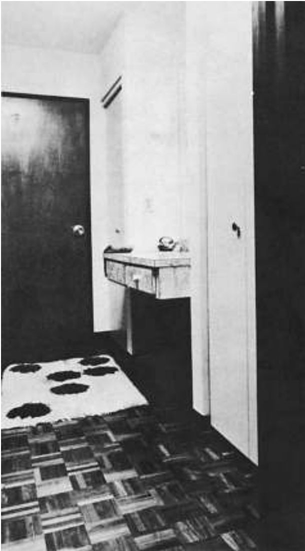
Figure 2-7 Wood-tile flooring. (Courtesy of United Gilsonite)
