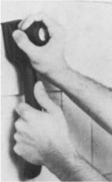
Figure 5-19 Scrape off all loose paint before painting.
