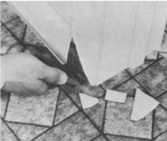
Figure 2-11 A utility knife is used to trim flooring. (Courtesy of
