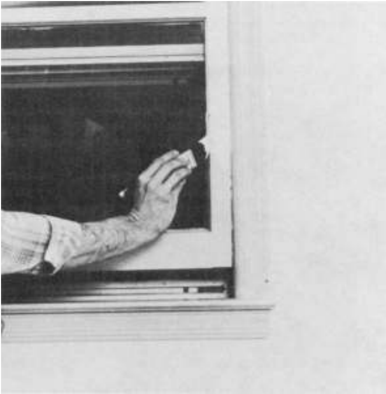
Figure 5-8 Painting window sash with brush at the angle shown makes the job easier.
