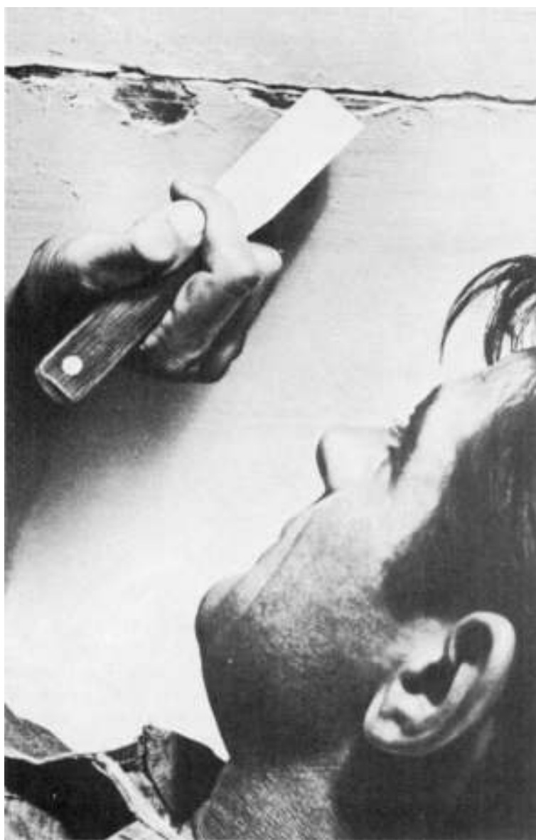
Figure 5-4 Patch and smooth before painting.
