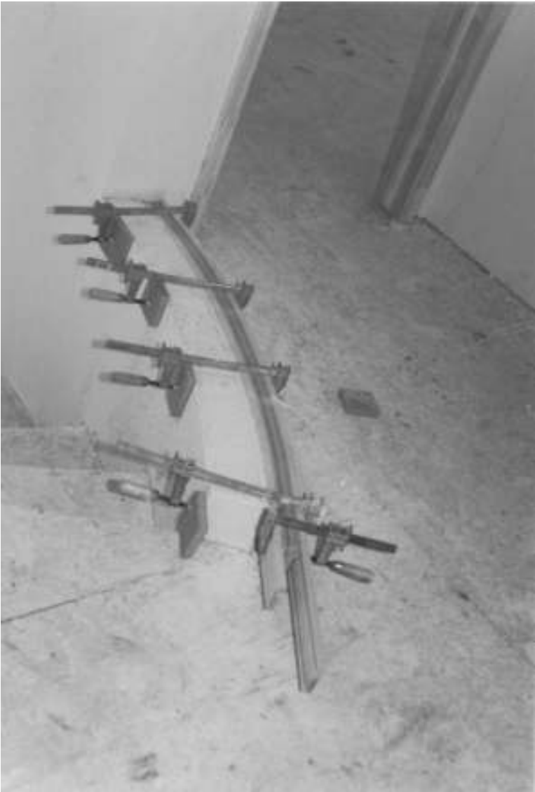
Figure I-23 First strips being held by clamps from the woodshop.
