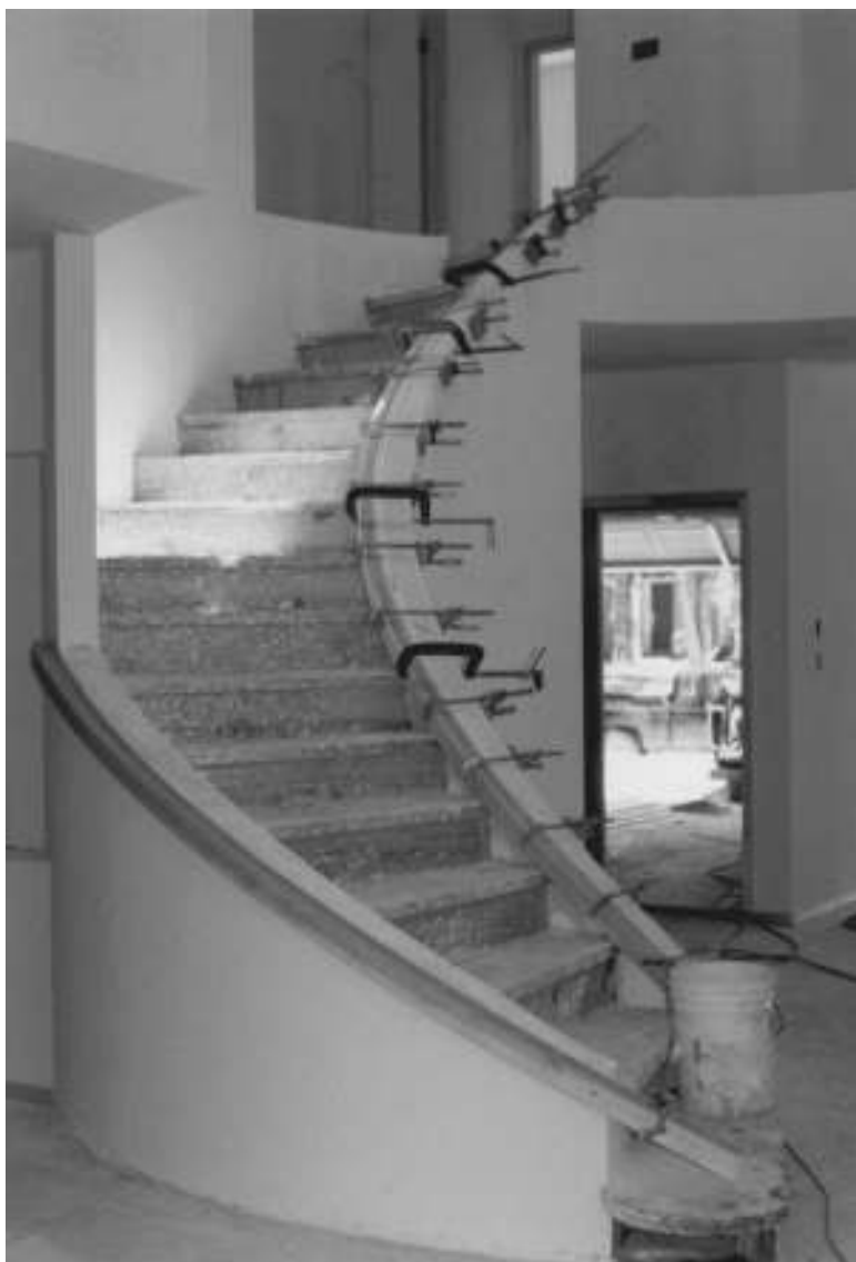
Figure I-28 Clamps holding the glued strips so they form the same curvature as the staircase.
