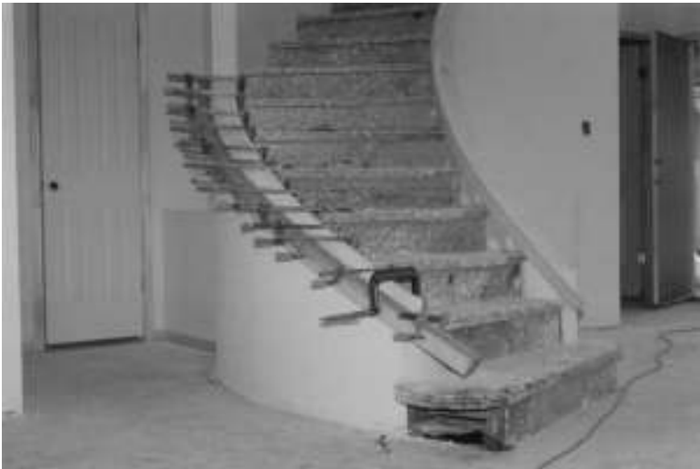
Figure 1-27 Clamps on the other and lower side of the staircase.
