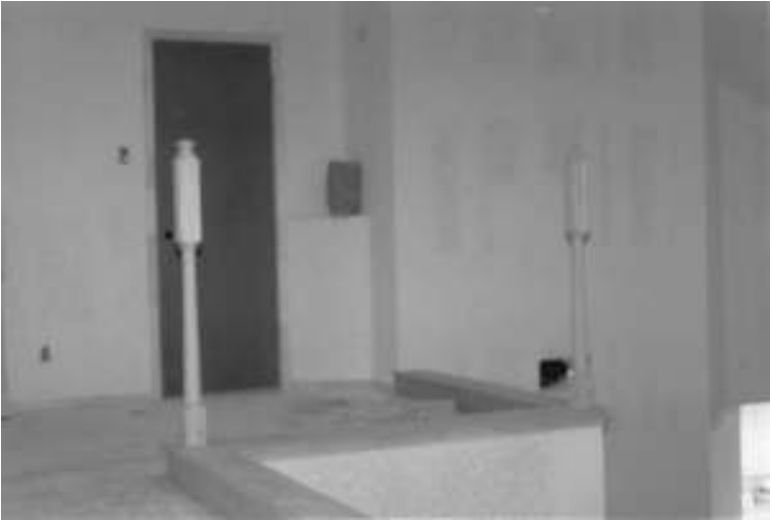
Figure I-30 Starting the installation of posts.
