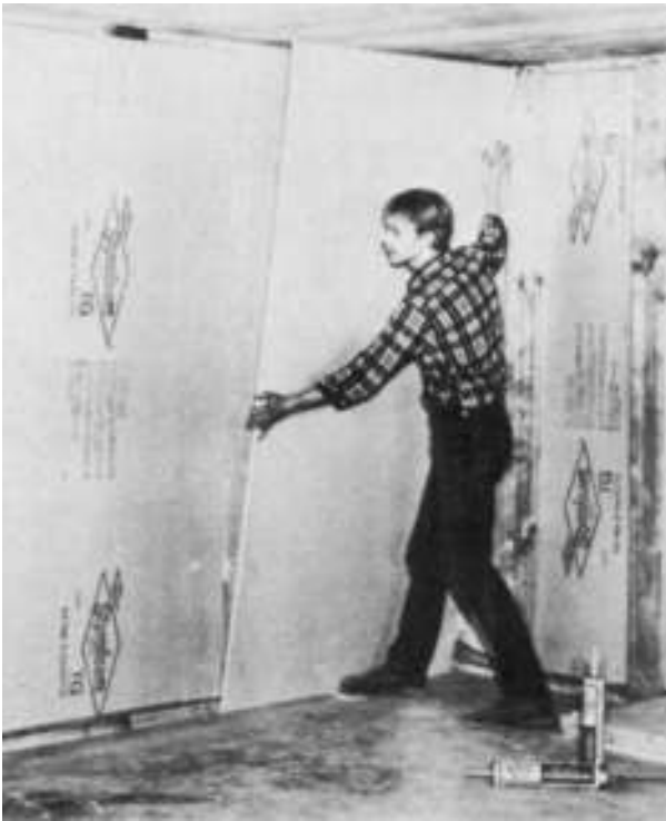
Figure 8-2 Material is glued on. Gypsum board must be used over plastic if material is combustible. (Courtesy of Certain-Teed)
