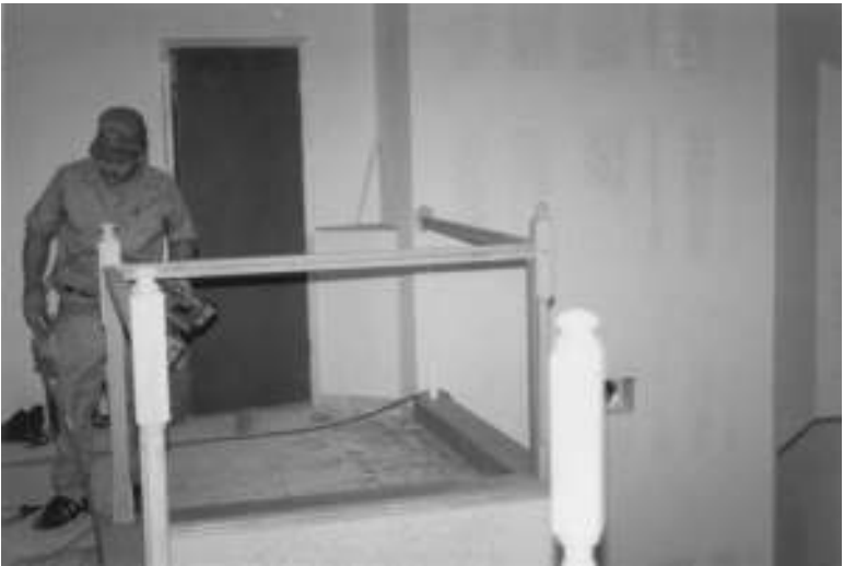
Figure I-31 First installation of the handrail.
