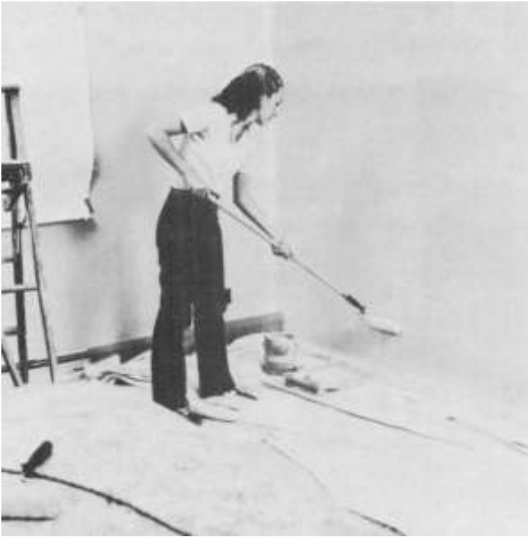
Figure 5-7 A long stick with a roller can make painting simpler. Do walls after ceiling. (Courtesy of Benjamin Moore)
