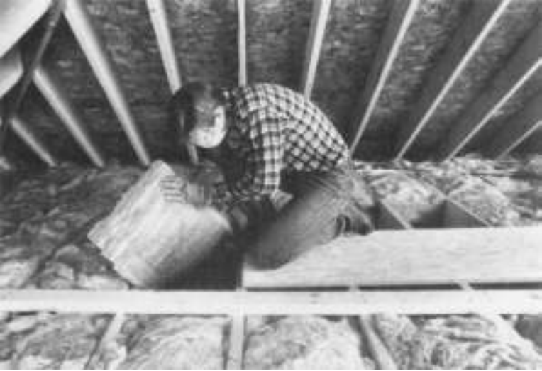
Figure 8-3 In the attic, blanket insulation fits between joists. Use plywood as temporary floor during installation. (Courtesy of Owens-Corning)
