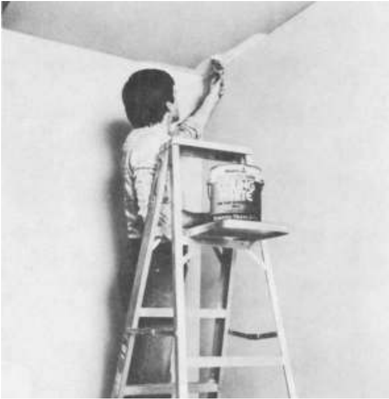
Figure 5-5 Cut in ceiling... (Courtesy of Benjamin Moore)
