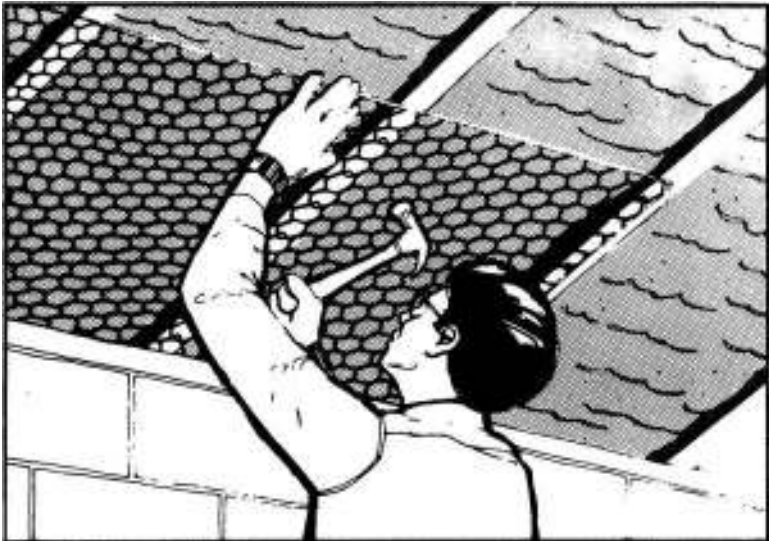
Figure 8-16 Floors above unheated spaces should be insulated. Wire netting can be used to retain material.
