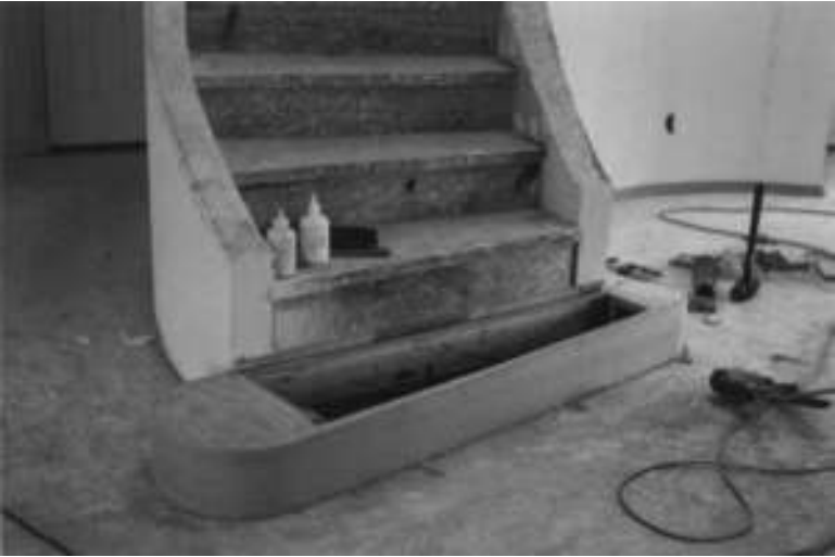
Figure 1-21 Close up view of the prefabricated last step coming down.
