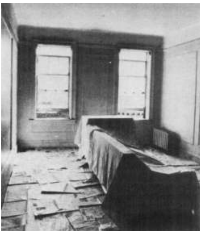
Figure 5-20 Moving furniture to room center and covering it up as shown is a good idea for an interior job.
