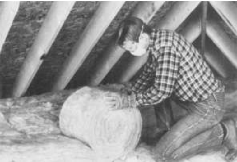
Figure 8-13 Additional insulation is added by laying a second layer of blankets or batts perpendicular to the first layer. (Courtesy of Owens-Corning)
