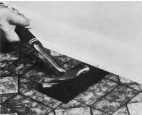
Figure 2-13 The final step is to reinstall molding. (Courtesy of Congoleum)
