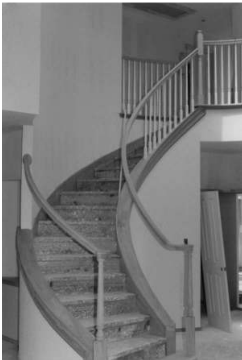
Figure 1-29 Handrails installed and installation of balusters progressing.
