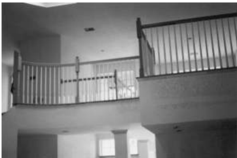
Figure I-33 Handrail and balusters in place.
