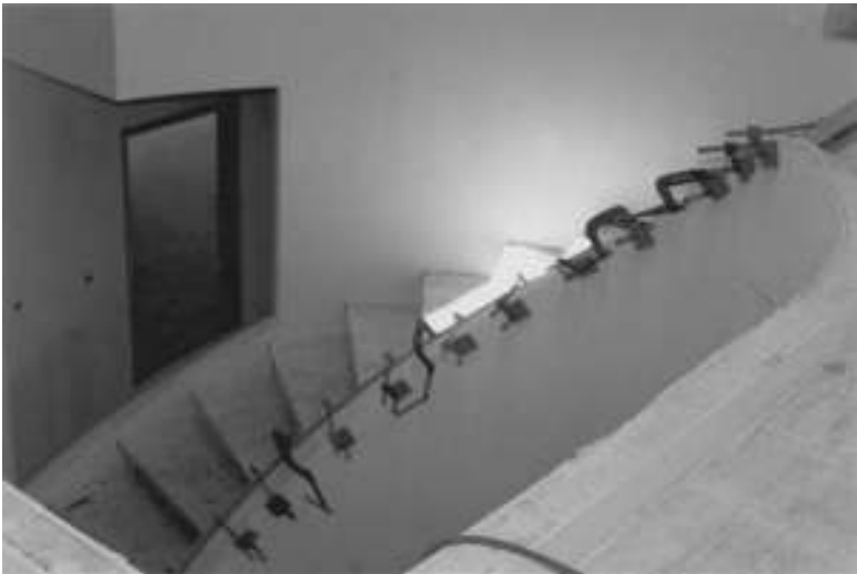
Figure 1-25 Clamps on the longest run of the gluing process.
